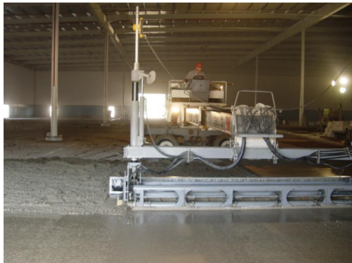
Figure 2-1: Levelling of the concrete floor with laser screed.
