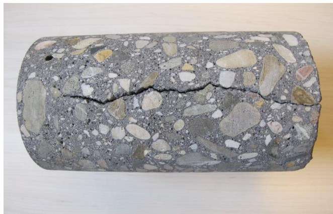
Figure 5-2: Crack due to shrinkage eliminated at the top surface.
