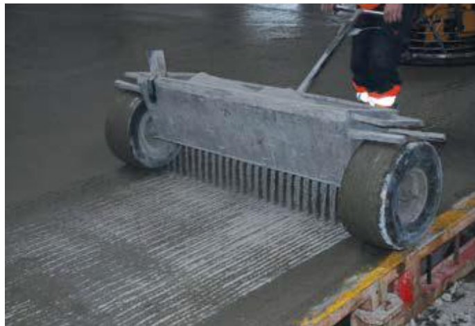
Figure 2-6: Spreading a mixture of cement and quartz using a distributor.
