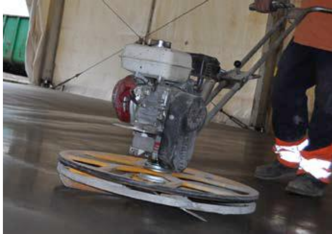
Figure 2-7: Power float fitted with angled blades for polishing.
