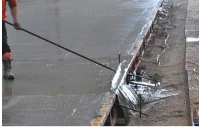
Figure 2-3: Elimination of the bleed water before starting the finishing operations.
