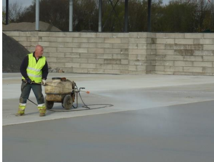
Figure 2-8: Spreading of a curing compounds.
