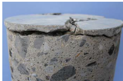
Figure 1-2: Concrete core with delamination.
