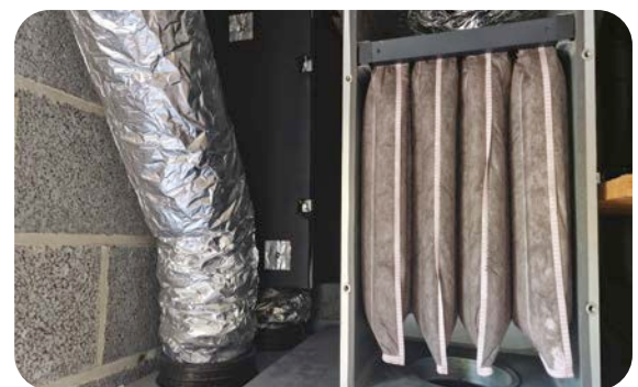
2 Bag filter in a filter box.
