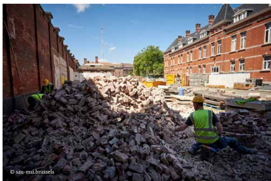
Usquare Brussel - demontage bakstenen
