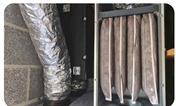
2 Bag filter in a filter box.
