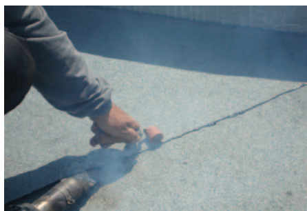
Afb. 3 Gelaste overlapping.
