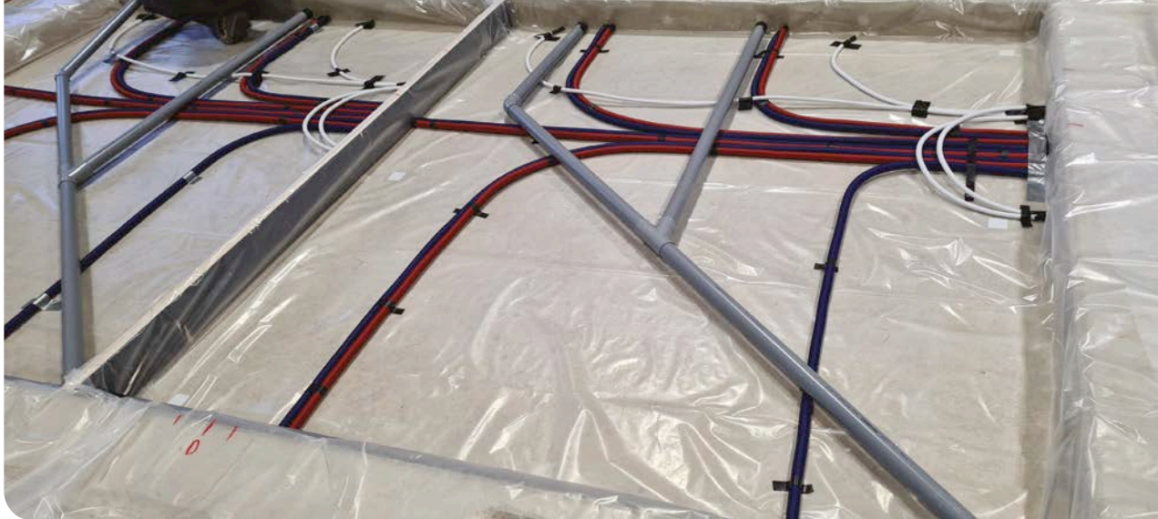
2 Two test setups with an identical pattern of pipes, before application of the filling layer.
