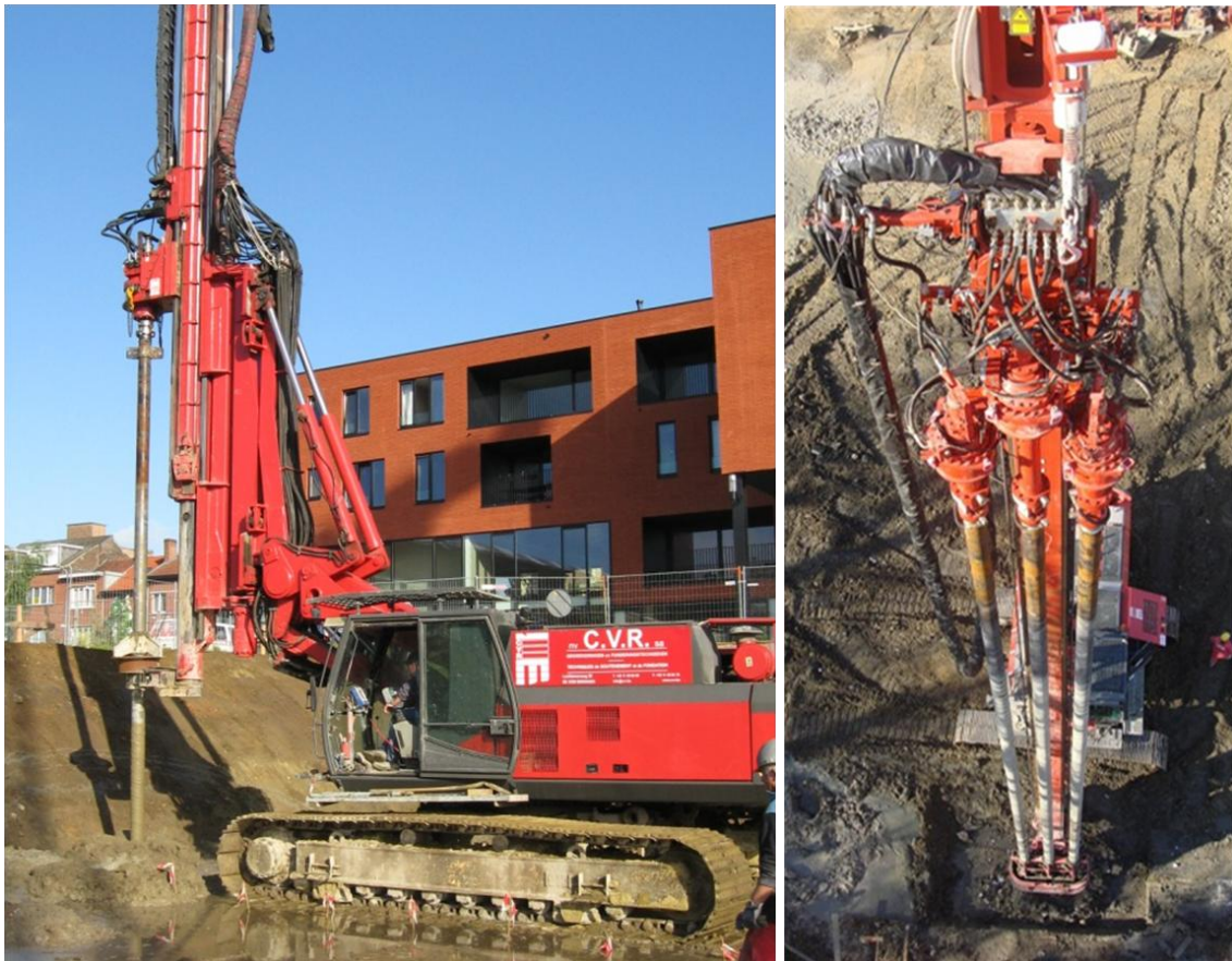
Figure 3: CVR C-mix ® machine and its Triple version
