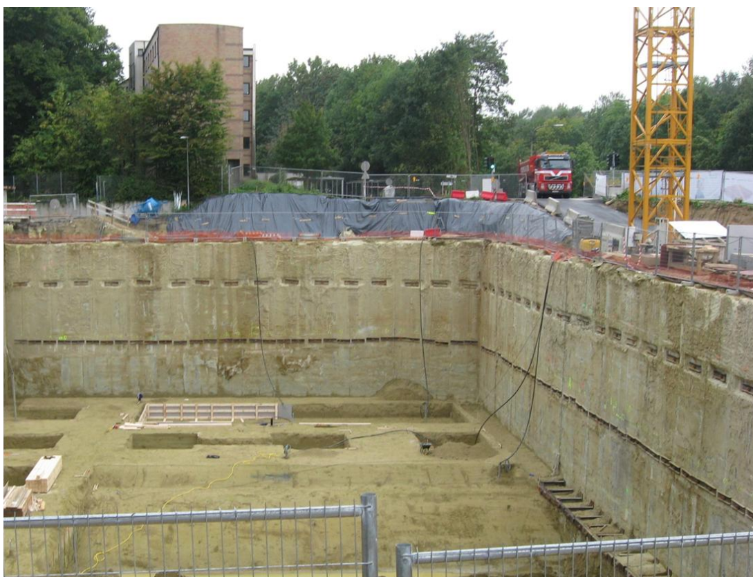
Figure 7: SMW performed with the CSM technique (Lameire Funderingstechnieken n. v.)
