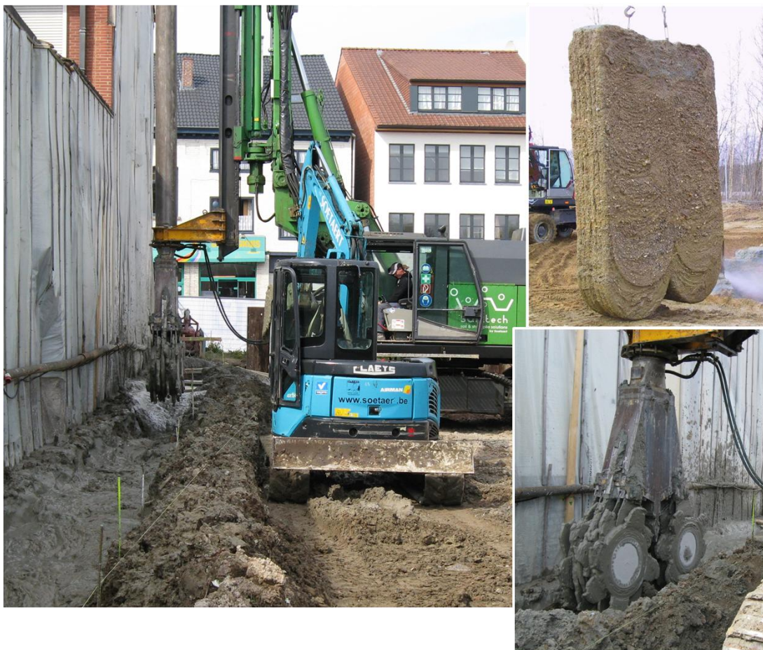
Figure 6: The cutting wheels of the CSM machine and the resulting CSM panel (Soetaert - Soiltech)
