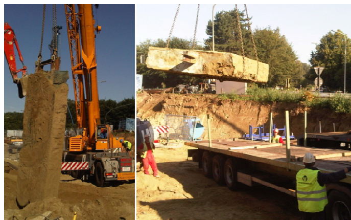
FIG. 4. Excavation and transportation of a real-scale soil mix panel (type CSM)
