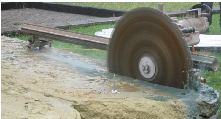
Figure 4: Sawing of a CSM panel
