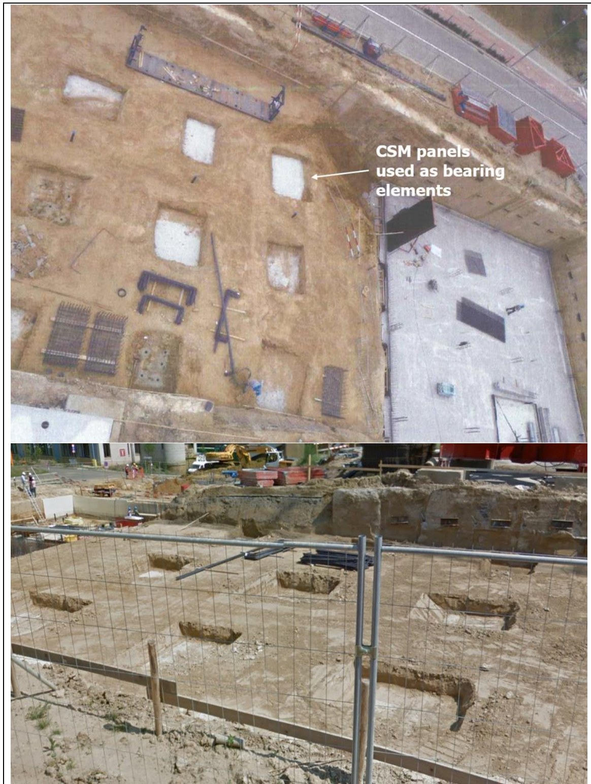
Figure 38: Different views of the CSM-panel caps after execution during summer 2013
