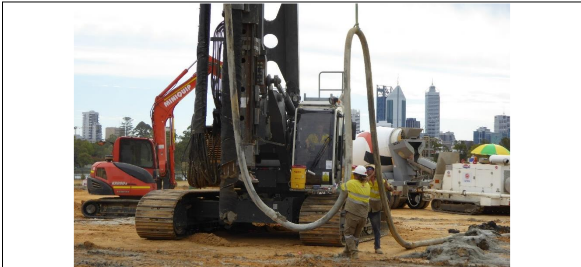
Figure 27: Photograph of a CMC auger
