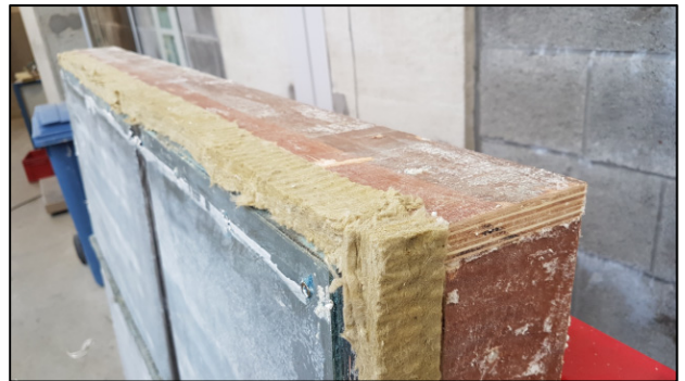
Figure 4. Pre-attached frame with a strip of mineral wool in front of it to avoid cold bridges.
