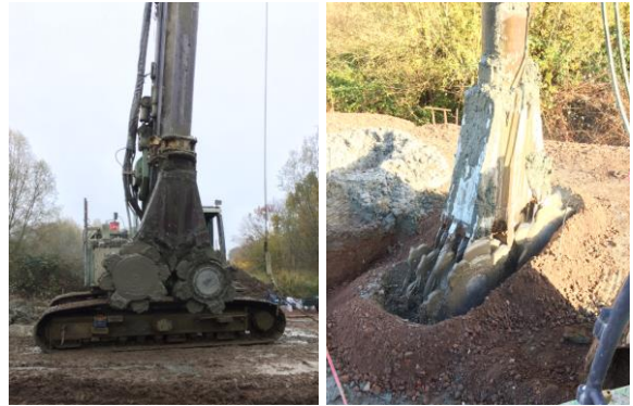
Figure 2. CSM machine and cutter on the test site of Melle
