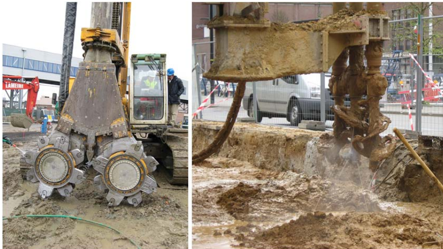
Figure 1. Illustration of typical deep mixing equipment in action on Belgian construction sites: Cutter Soil Mix (CSM) system of Bauer (left) and triple shaft configuration TSM system of Smet F&C (right).
