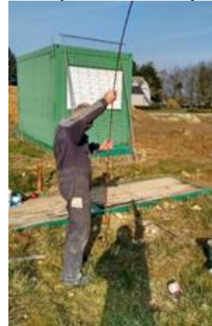
Figure 5. Optical fiber sensors installation
