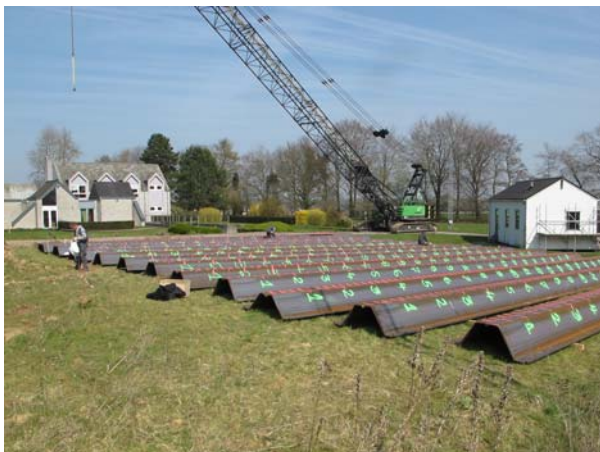
Figure 2. Marking of the double sheet piles before installation
