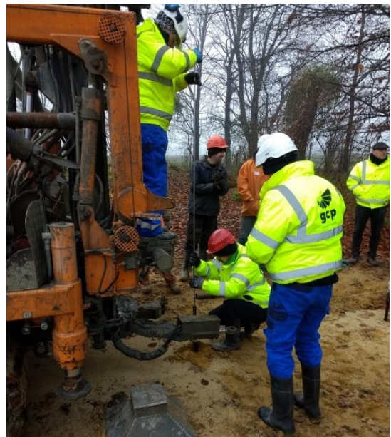
Figure 5. Installation of the injection tube inside the hollow steel bar
