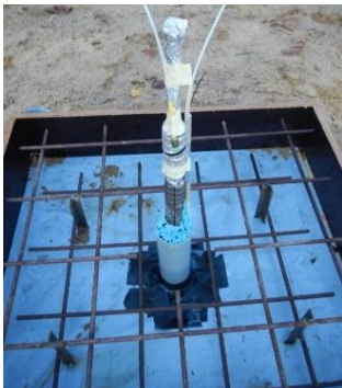
Figure 6. Isolation of the steel bar with the PU foam
