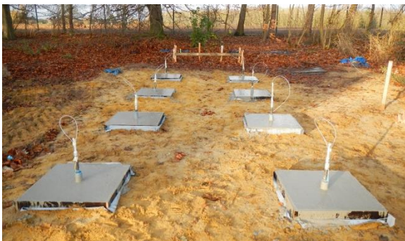
Figure 7. Test location after concreting the eight slabs
