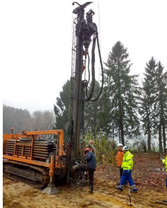
Figure 4. Dry drilling of the steel bars into the ground
