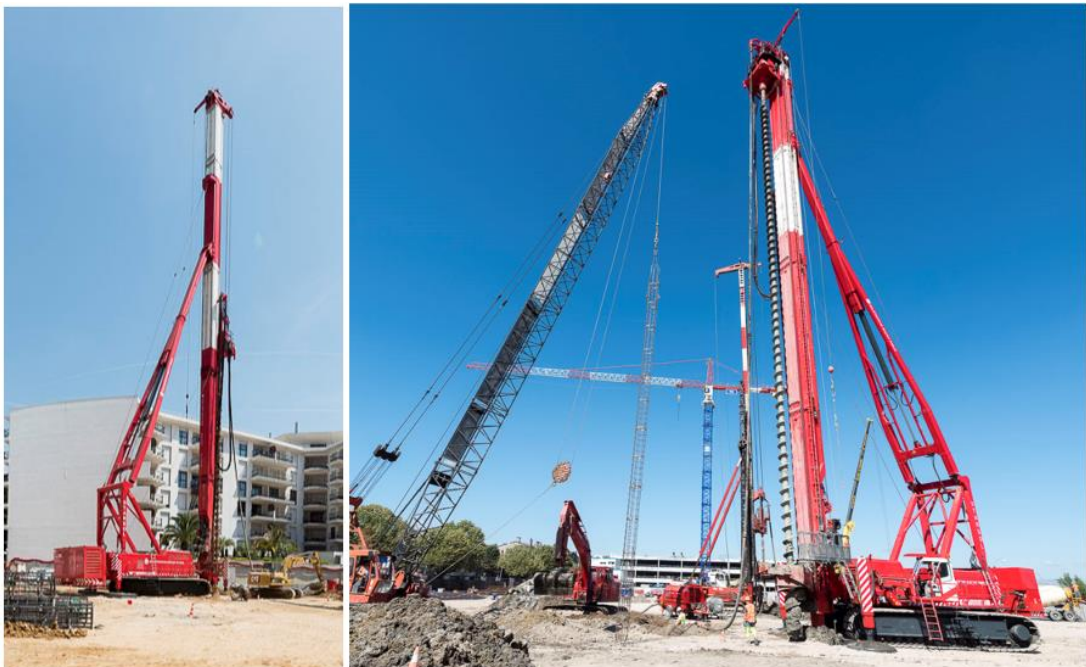
Figure 7. Soletanche-Bachy Starsol rig F5000
