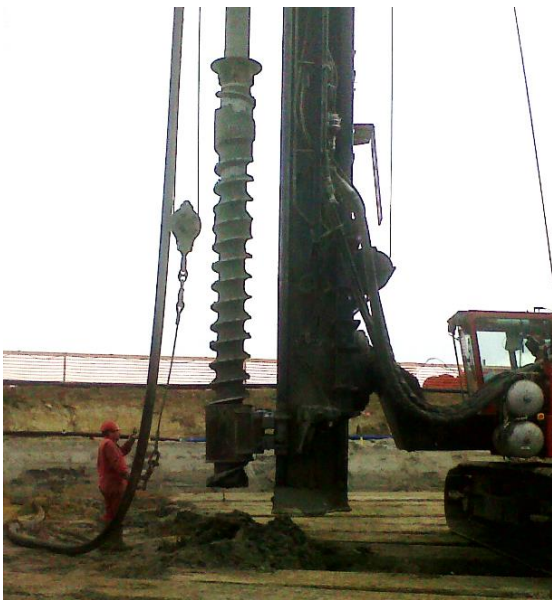
Figure 12. Screw pile with oversized portion of excavation auger at the bottom (Bottiau, 2014)
