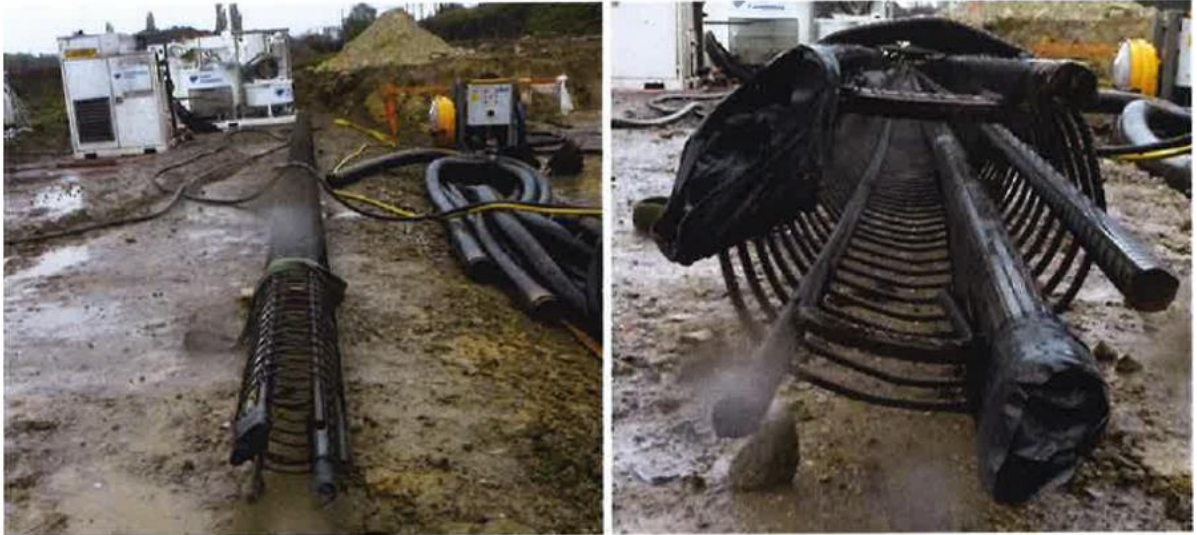
Figure 14. Haren test site - Illustration of the reinforcement cage provide with reservation tubes for the extensometer system
