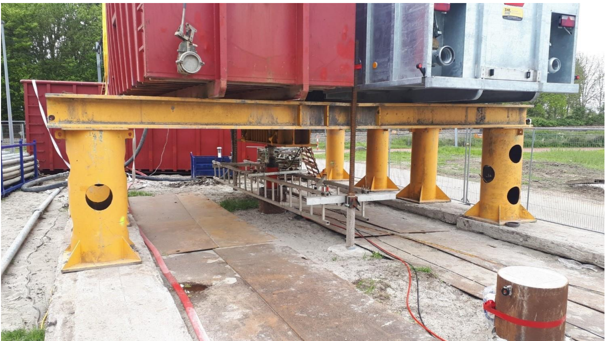
Figure 23. Set up of the compressive load test on a micropile
