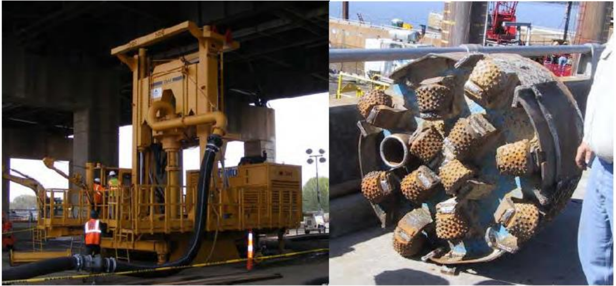
Figure 25. Reverse Circulation Drilling – limited headroom and full face drilling tool (Brown , 2012)
