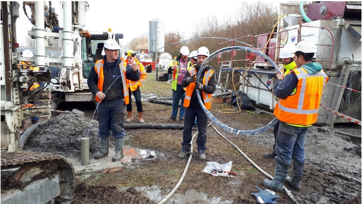
Figure 22. Installation of the instrumentation in a 67m deep micropile
