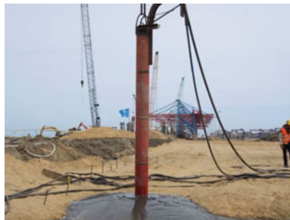
Photo 2: Operation of vibro-compaction in action
