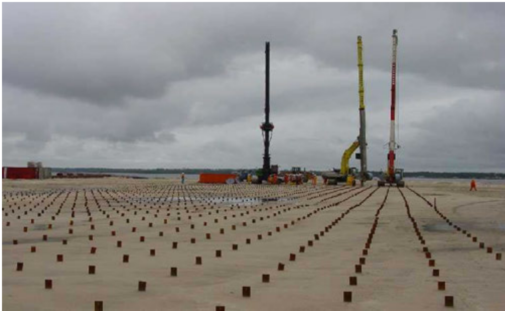
Photo 1: Installation of Deep Vertical Drains. Situation before Intermediate Drains in the Upper Clay are Installed down to the Middle Sand (CASE 1).
