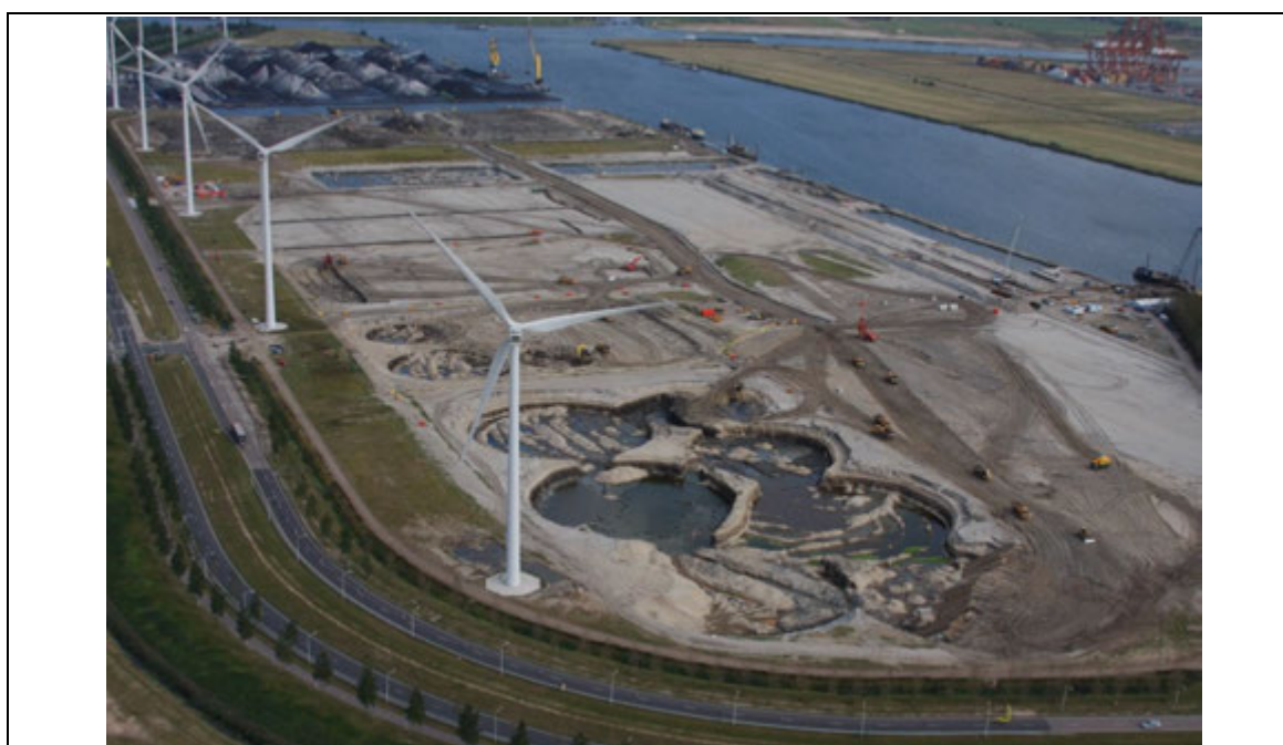
Photo 3: aerial overview of the project with the different phases
