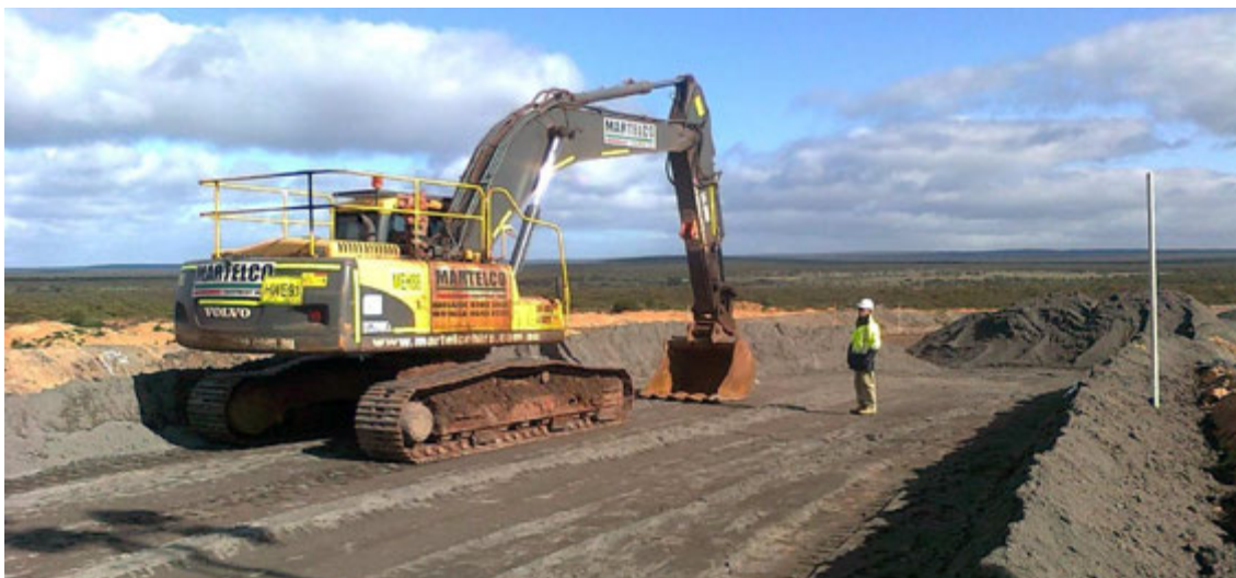
Photo 2: Test pad construction showing excavator used.
