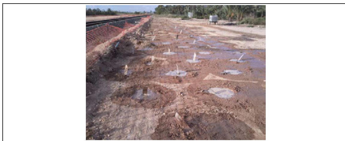
Photo 1: Treatment by vertical drains.
