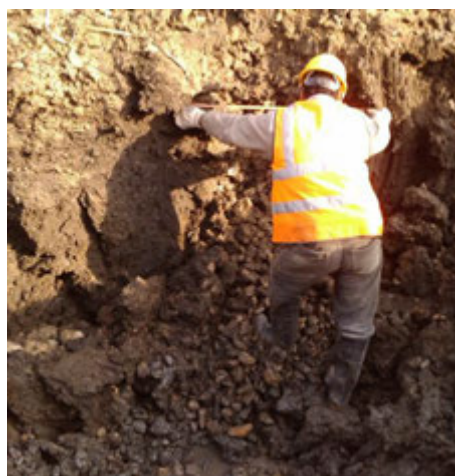
Photo 4 : Excavated stone column 2 weeks after construction
