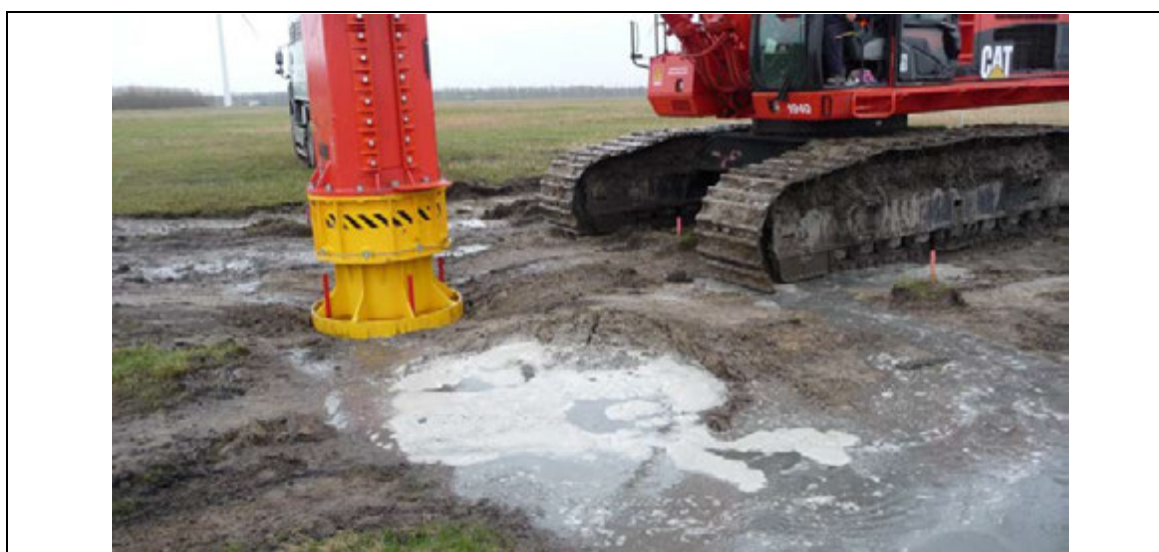
Photo 1: Compaction of a trial location. Note the subsidence on the surface and the water in the previously compacted location
