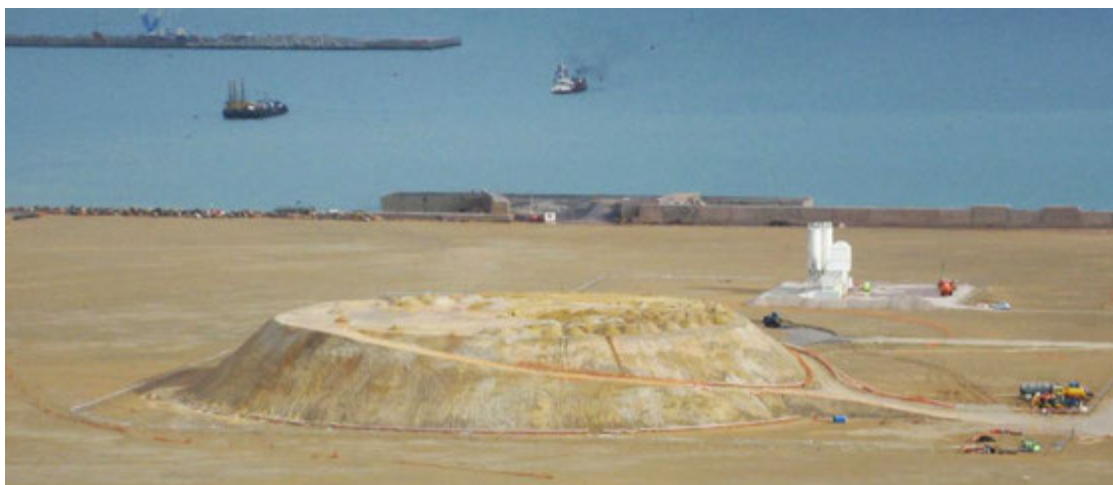
Photo 2: Completed Preload of Tank Nr 1
