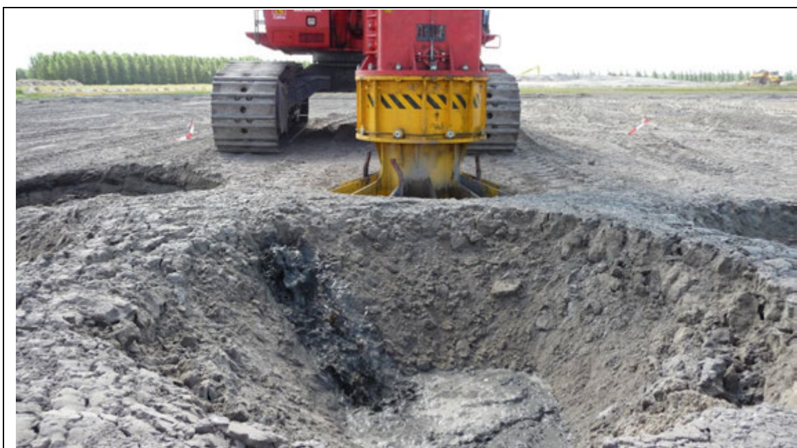
Photo 4: excess pore water escaping to the surface during the compaction
