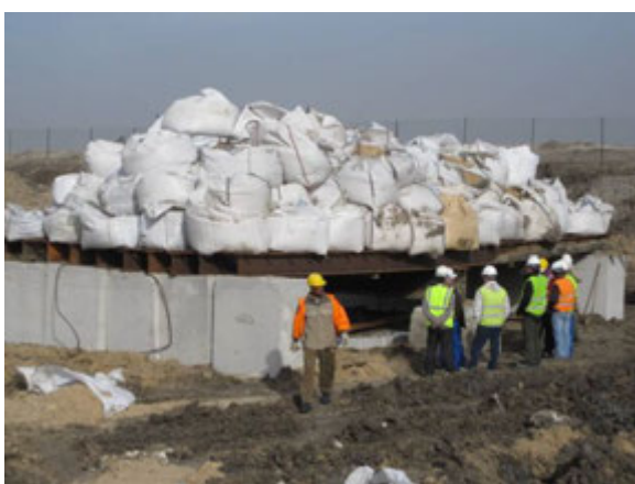
Photo 3 : Excessive vertical displacement of the improved ground during plate load test
