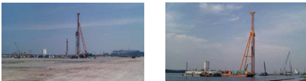
Figure 1.1 DM on-land rig and off-shore barge in Vietnam
