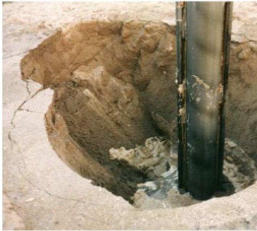
Figure 6: Crater due to execution
