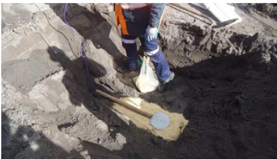
Photo 3: Preparing the EPCs in situ on bedding sand.
