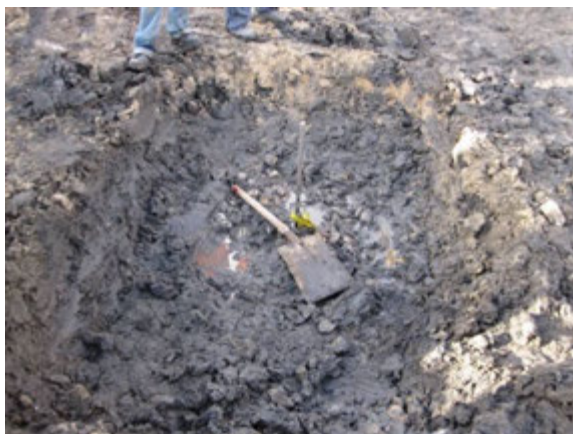
Photo 1 : Water logging of stone column
