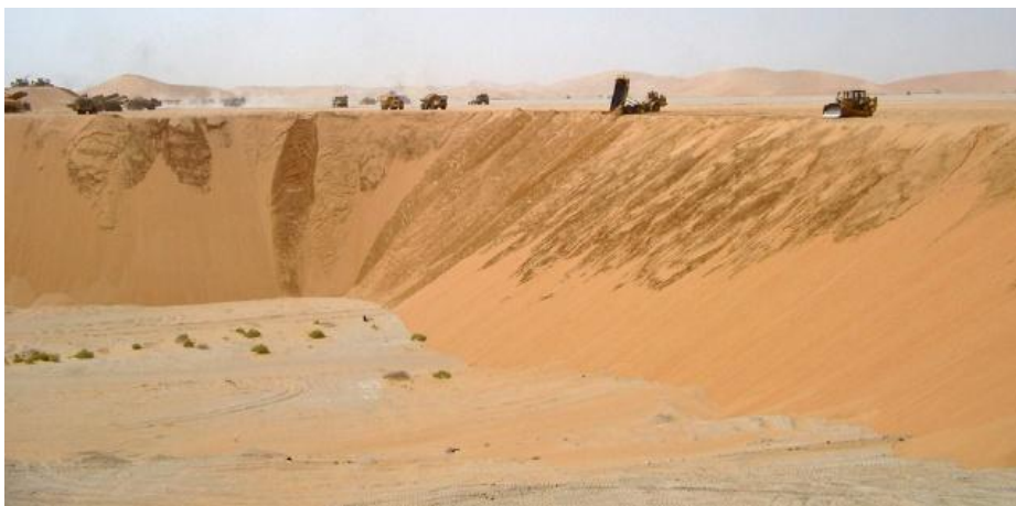
Figure 2: Backfilling and construction of the working platform by dumping
