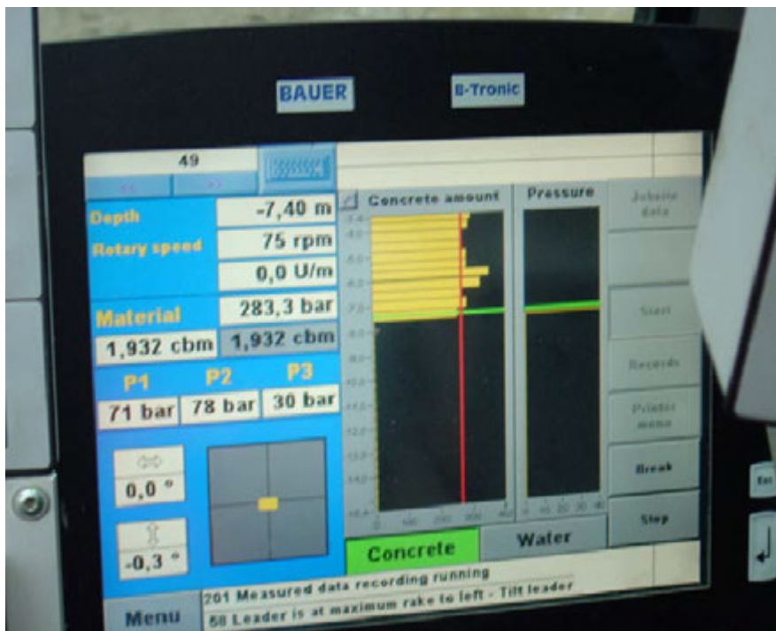
Figure 11: QC monitoring of grout flow rates, injection volume and pressure and penetration rate during execution of CSM wall (photo with courtesy of Malcolm Drilling Company)
