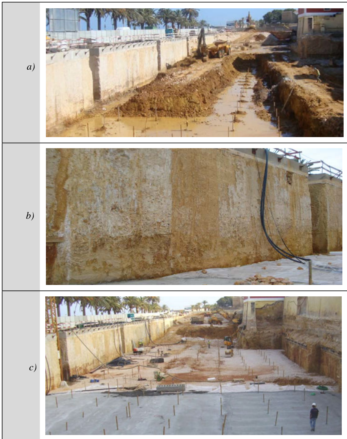
Figure 9: Views of the work during the excavation: a) excavation of 6 m depth; b) detail of the CSM wall; c) regularization of the bottom of the excavation.
