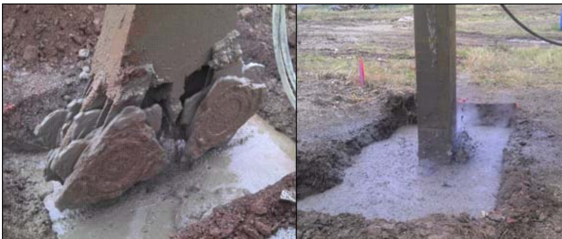
Figure 9: Execution of a CSM panel.
