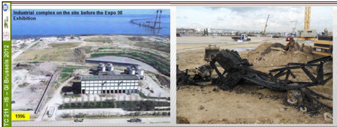
Figure 4: View of the previous industrial complex located on the site and example of the demolished waste found inside the heterogeneous landfill.
