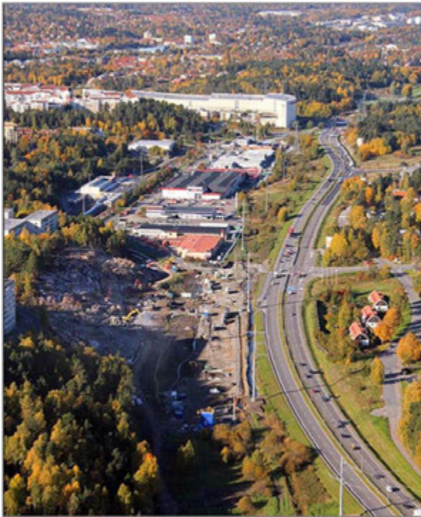
Photo 3: Jobsite Stockholm for the lime cement columns
