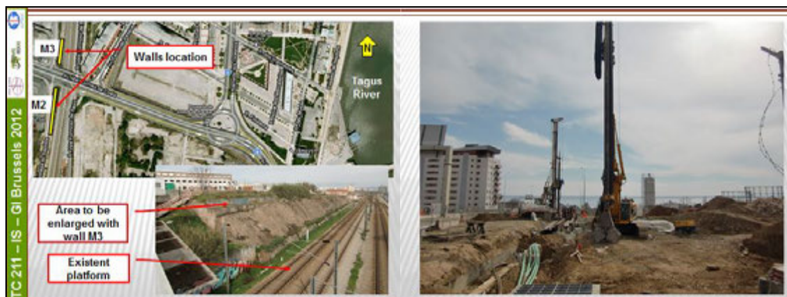
Figure 9: Site location and execution of the CSM panels at wall M2.
