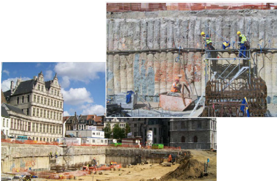
Figure 5: SMW performed with the help of the triple version of TSM (SMET-F&C)
