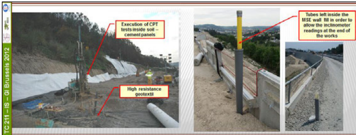
Figure 29: CPT tests at the “Marão” Motorway M4B wall base.
