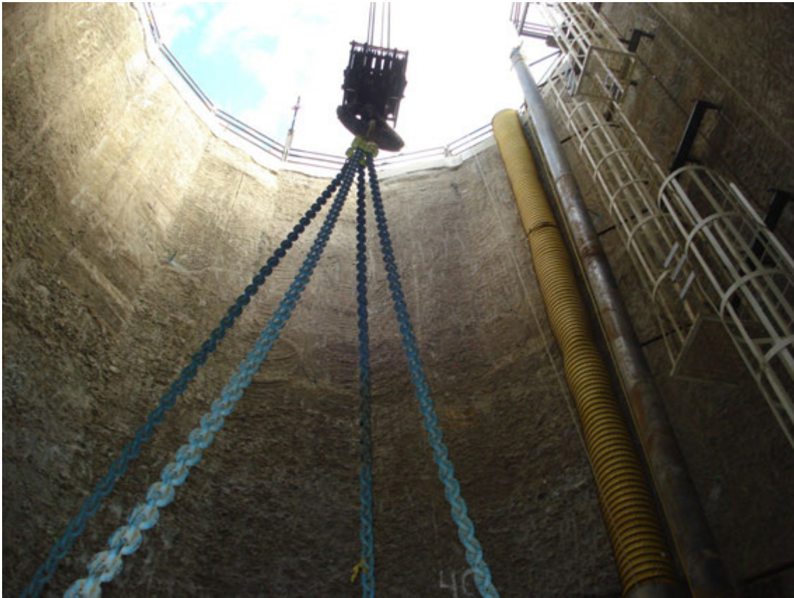
Photo 7: Excavated shaft L, excavation depth about 22 m
