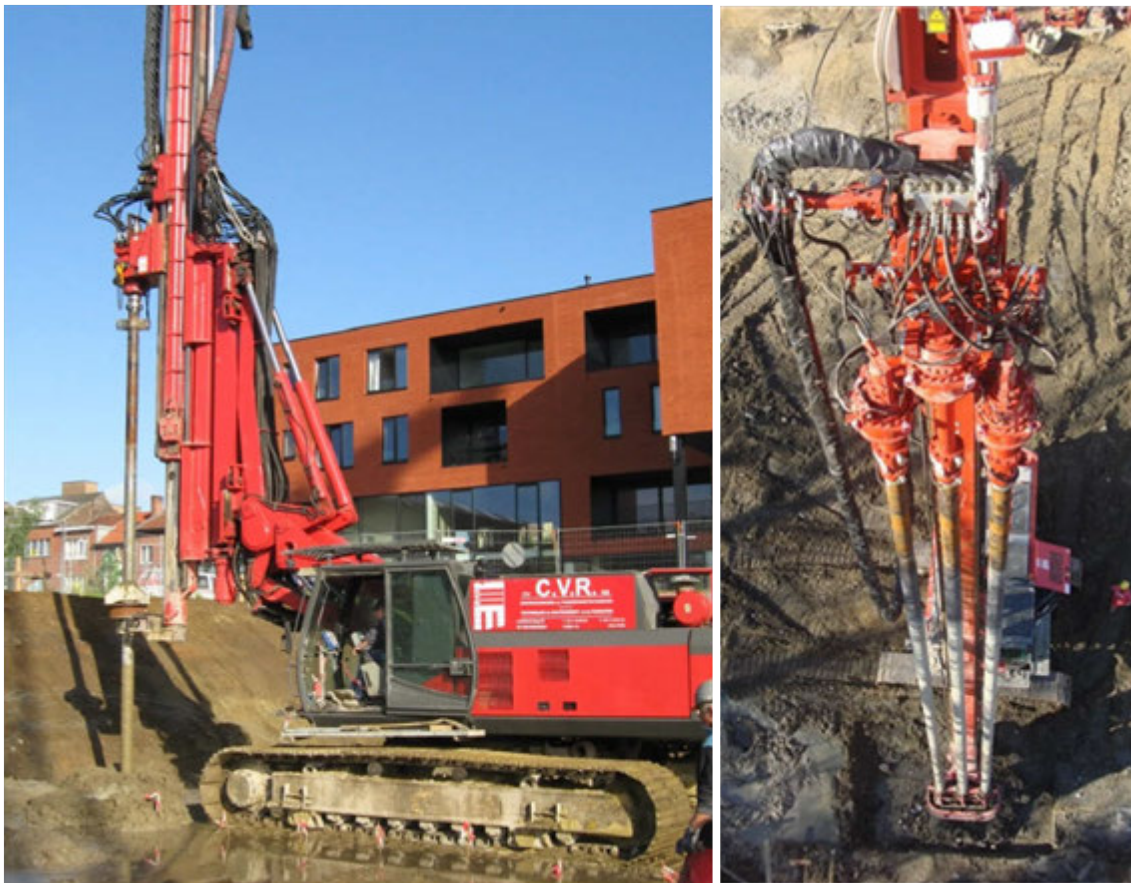
Figure 3: CVR C-mix ® machine and its Triple version
