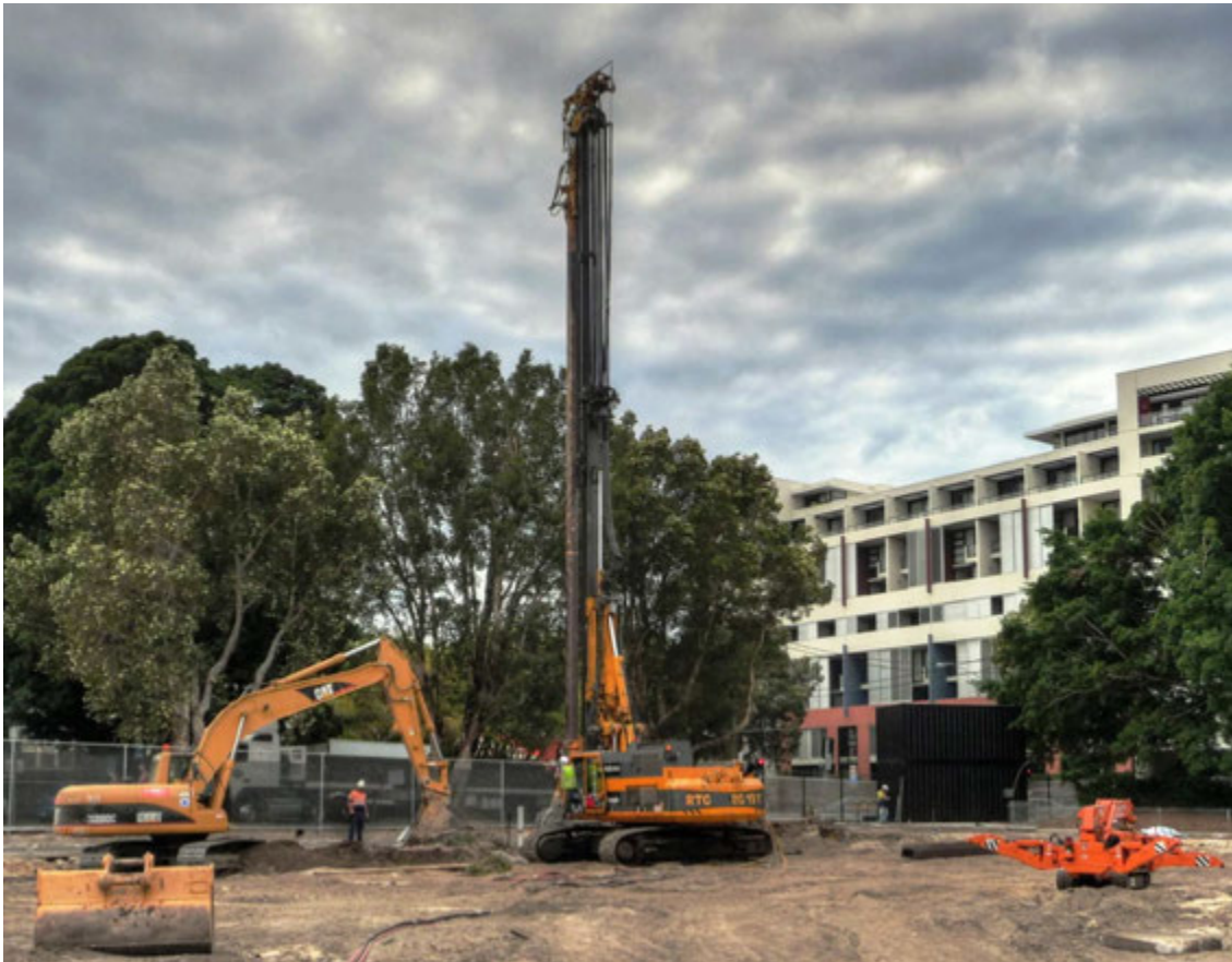
Photo 5: RTG RG 19 T and excavator for pre-excitation and backflow handling
