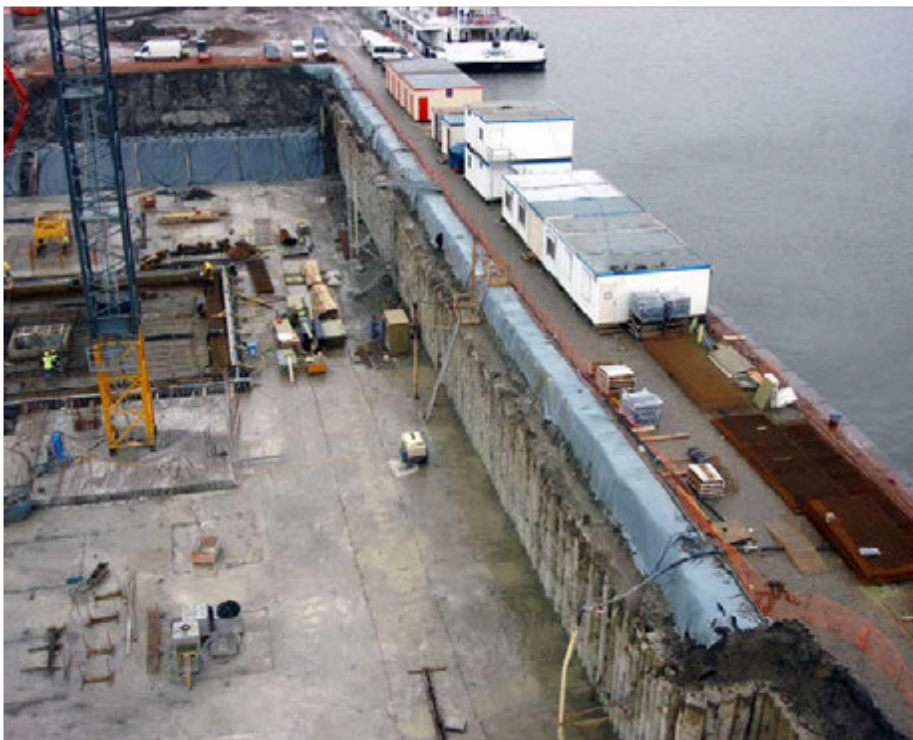
Figure 1: SMW with ground and water retaining functions
