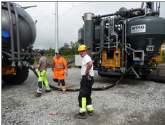
Photo 6: Filling procedure using a dumper
