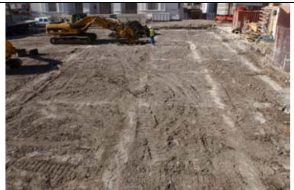
Photo 3 :Platform after execution of works
