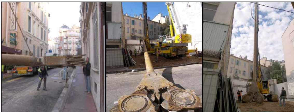
Figure 4: Installation of the equipment.
