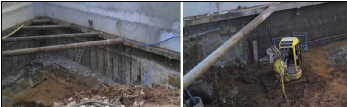
Figure 12: Partial views of the steel pipe struts.
