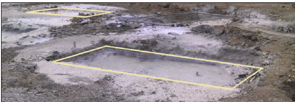
Figure 5: View of some panel caps..
