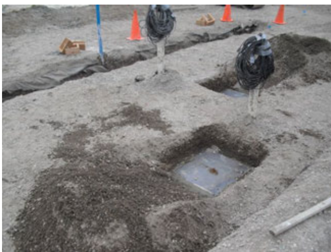
Figure 9: Installation of the Instruments
