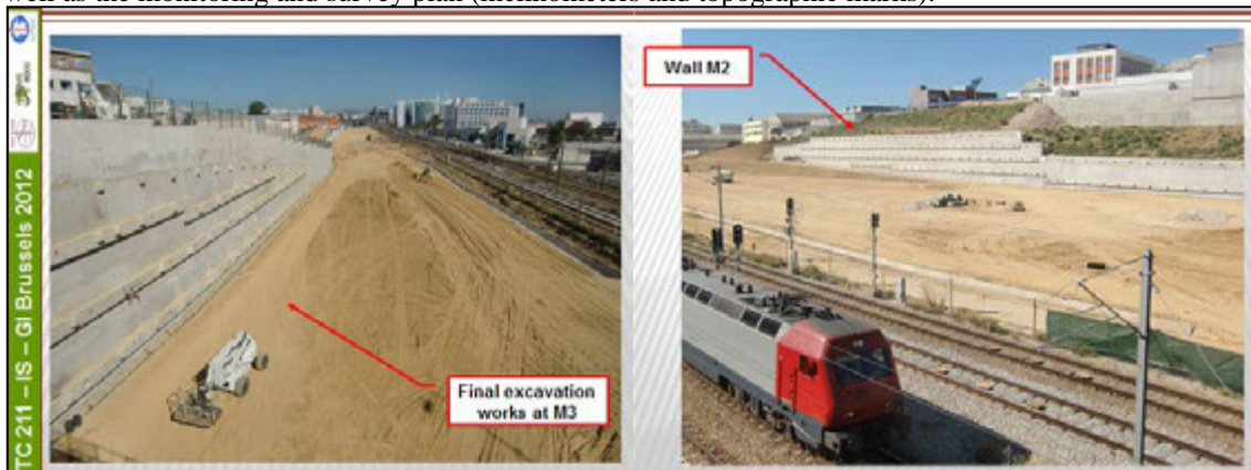
Figure 15: Views of the walls after the conclusion of the excavation works.
