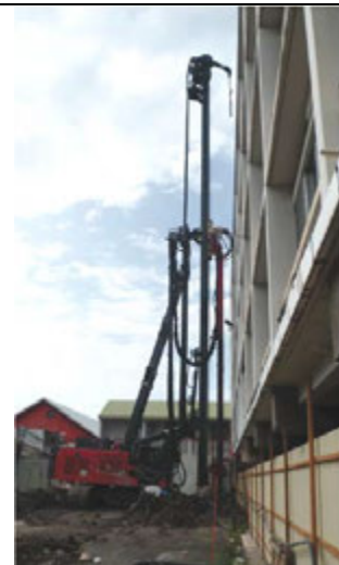
Photo 5 :Construction of panels close to existing buildings
