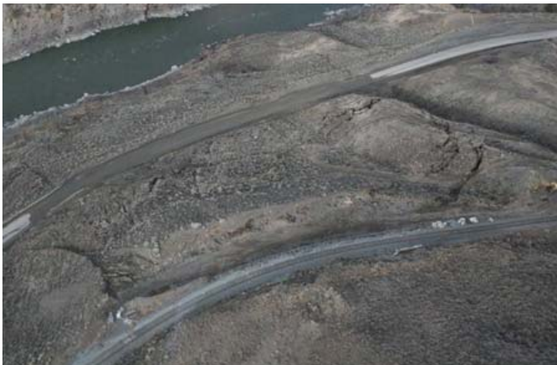
Figure 3: Aerial view of slide - October 2009: 1
