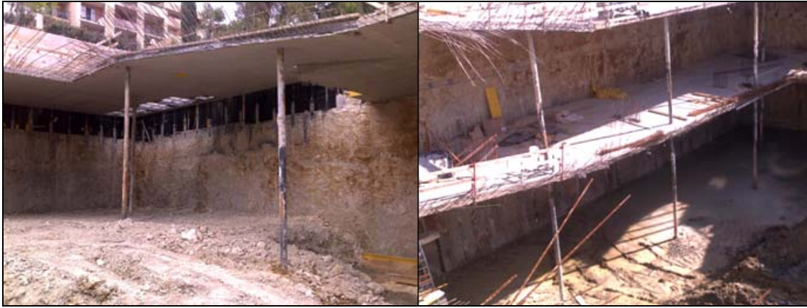
Figure 11: View of the work during the second level of excavation (on the left) and after the execution of the second level of slab bands (on the right).
