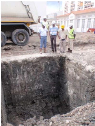
Photo 4 :Excavated caisson
