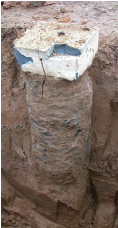
Figure 3: Excavation of column P2
