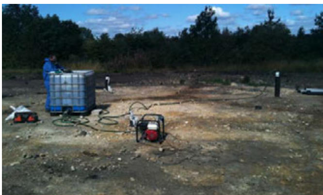
Figure 9: Pumping from one of the PRB walls.
