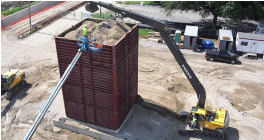
Figure 8: Picture of the construction of the Load Test Area (Form Work)
