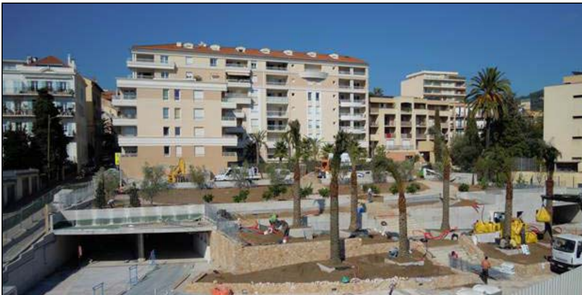
Figure 12: General aspect in the final phase of the work.
