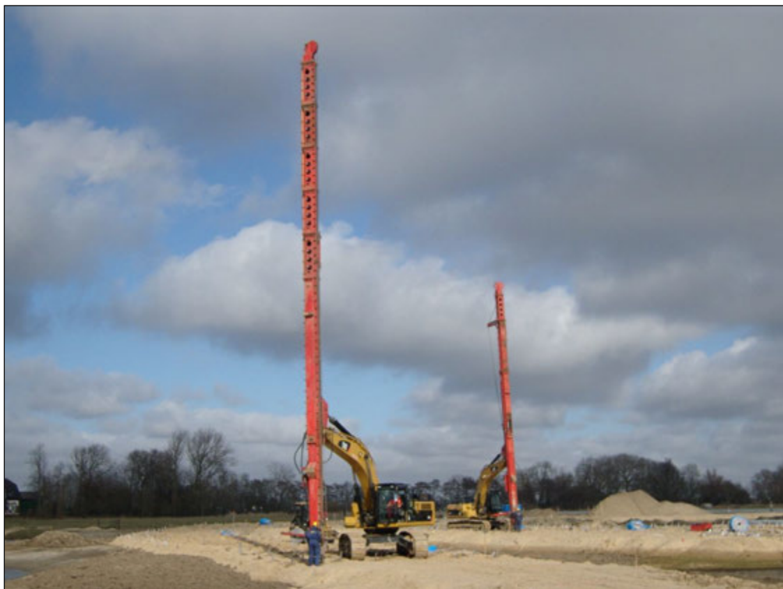
Photo 1: installation of vertical drains on a dry one meter thick sandplatform
