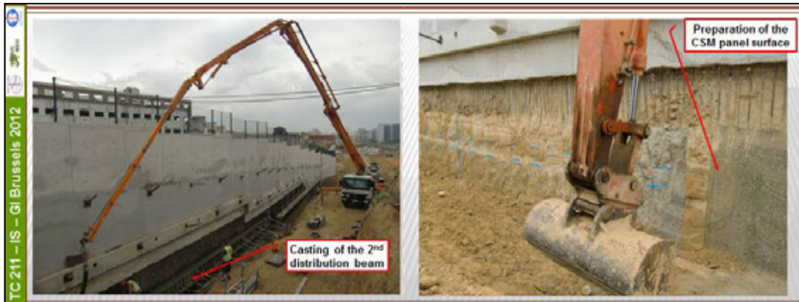
Figure 14: Views of the excavation works.
