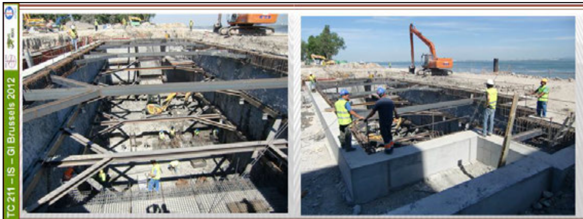
Figure 20: Views of the internal structure construction.
