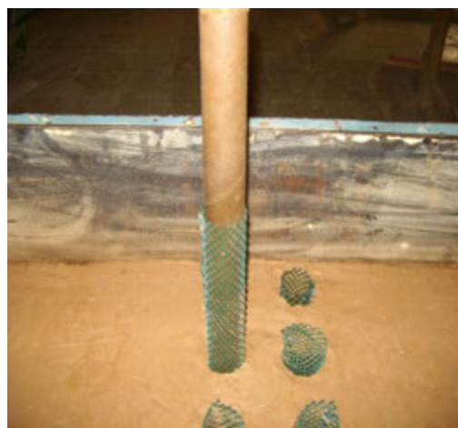
Photo 2: Construction of encased stone columns
