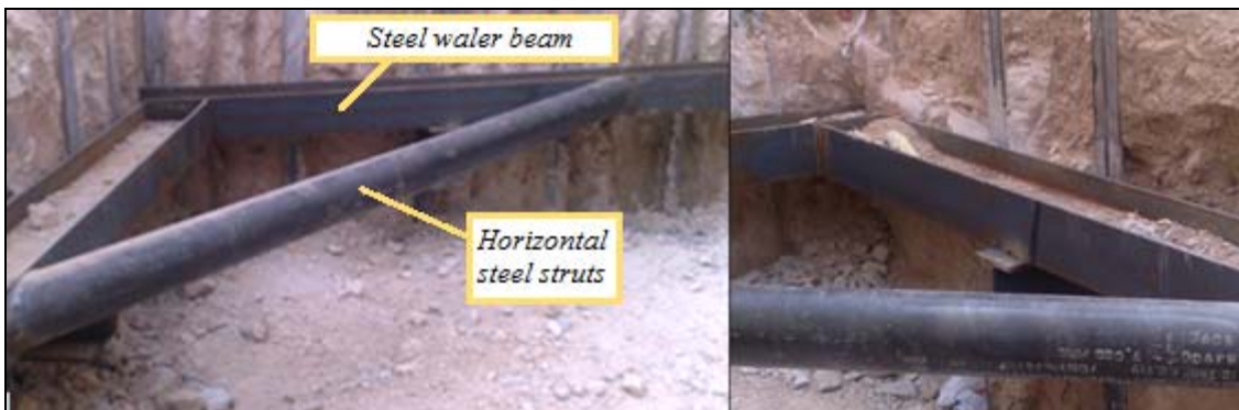
Figure 11: Detail of the steel waler beams connected to the pipe struts.
