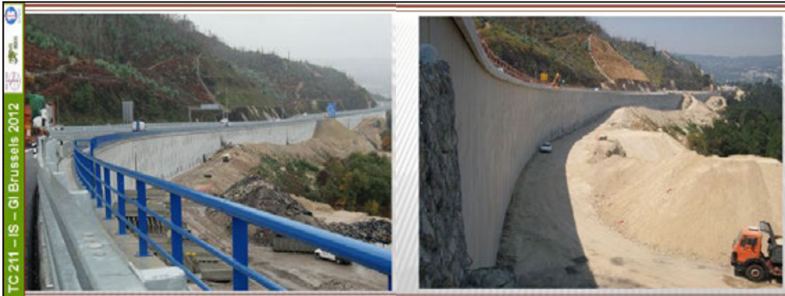
Figure 26: Views of the wall at the end of the works.
