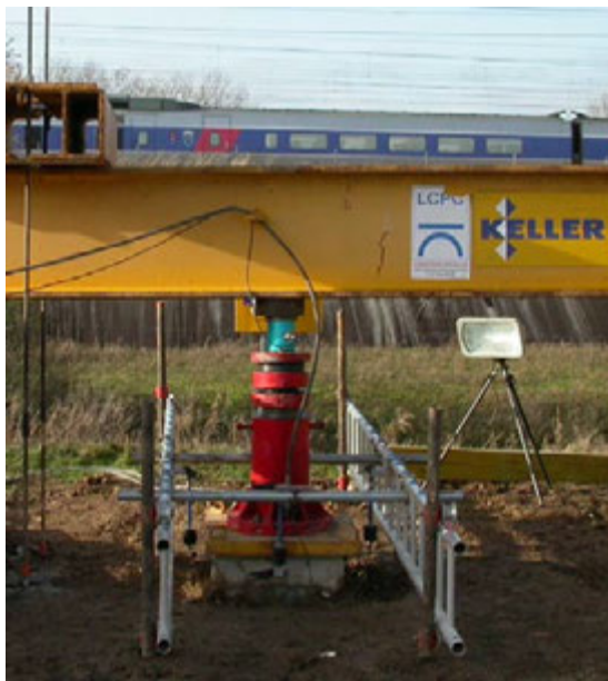
Figure 6: View of the load test system
