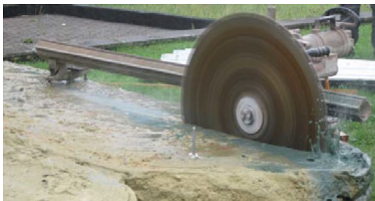
Figure 4: Sawing of a CSM panel
