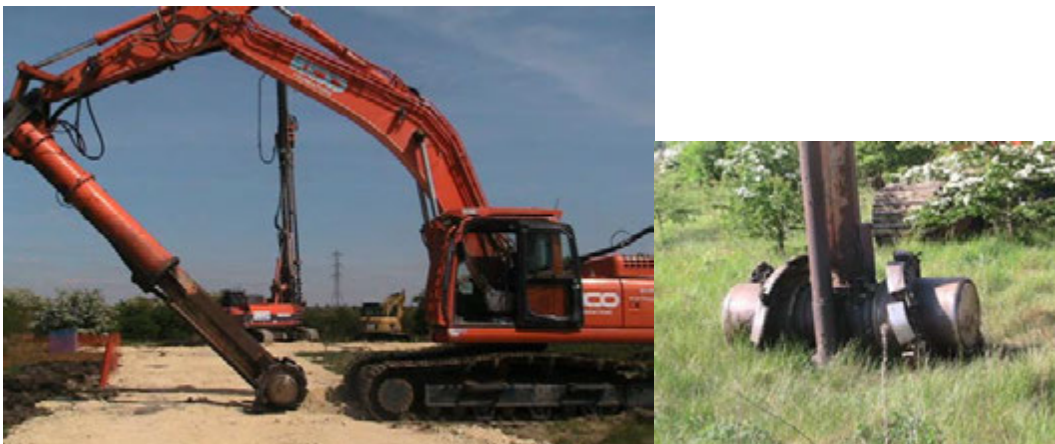
Figure 2: The ALLU system used in the ground improvement treatment sections
