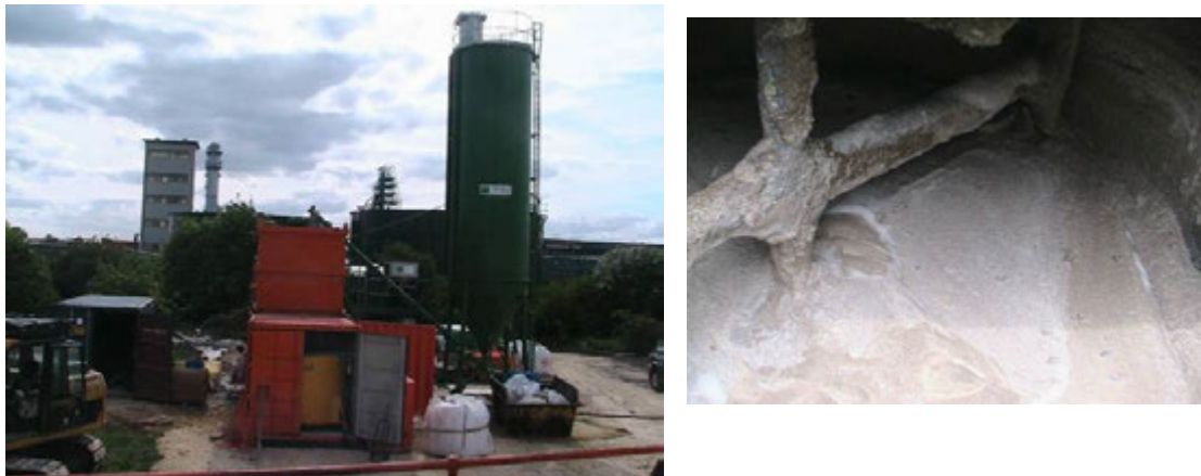
Figure 4: The batching plant and materials storage on site
