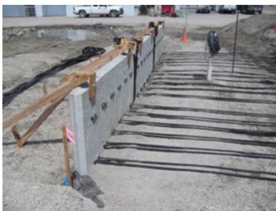
Figure 11: Installation of the MSE Ring Wall (Reinforced Earth Omega System)
