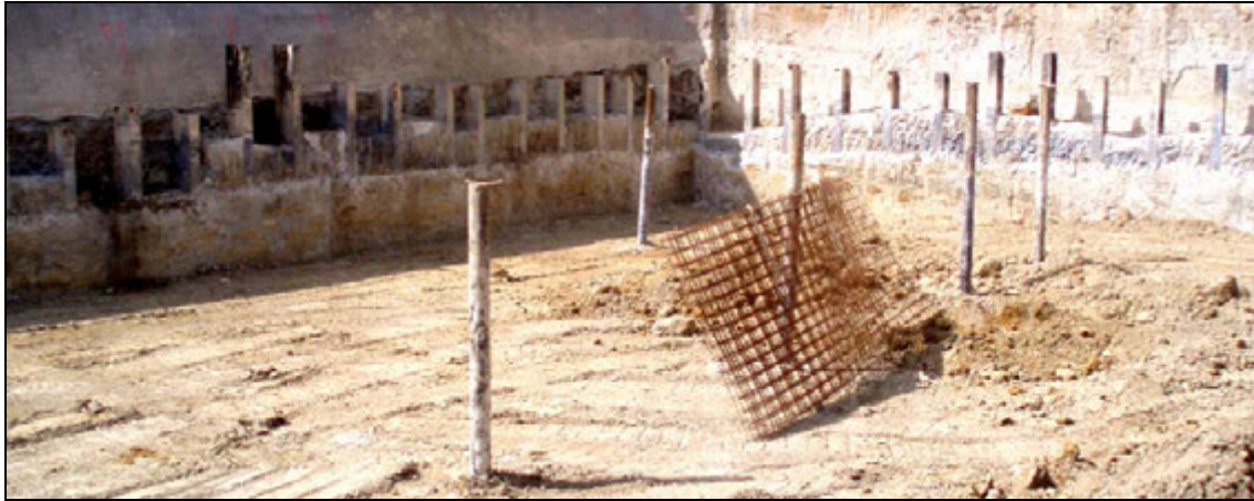
Figure 9: Foundation micropiles to the temporary support of the slab bands.
