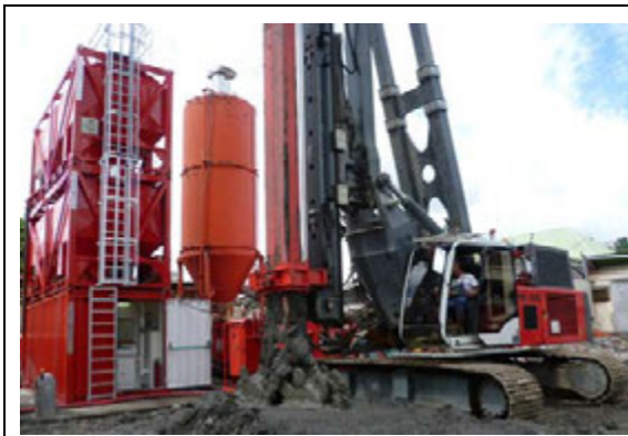
Photo 2 :CSM Equipment on LRB155
