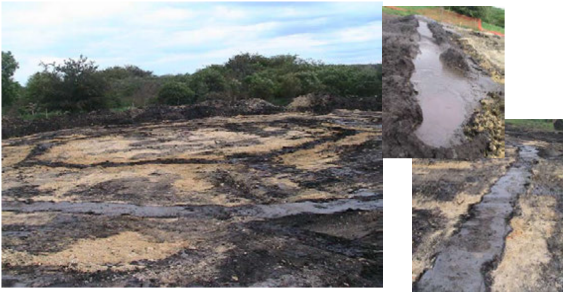
Figure 7: The hexagon set up with 6 inner PRB wall sections and 6 outer low permeability walls.
