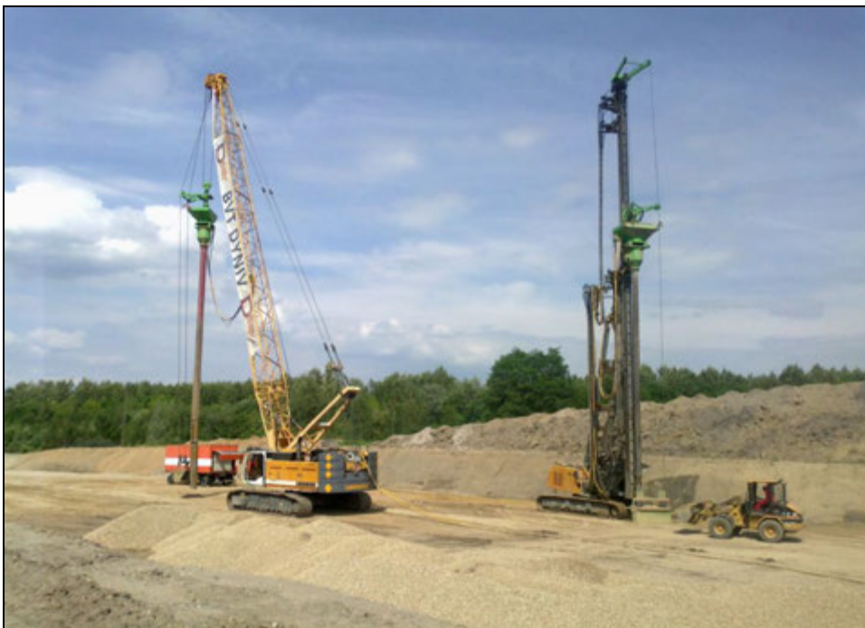
Photo 3: Leader-guided and free-riding-on-the-device technology for stone columns B176
