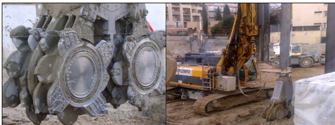
Figure 3: Detail of the cutting wheels (on the left) and general aspect of the hydromill (on the right).
