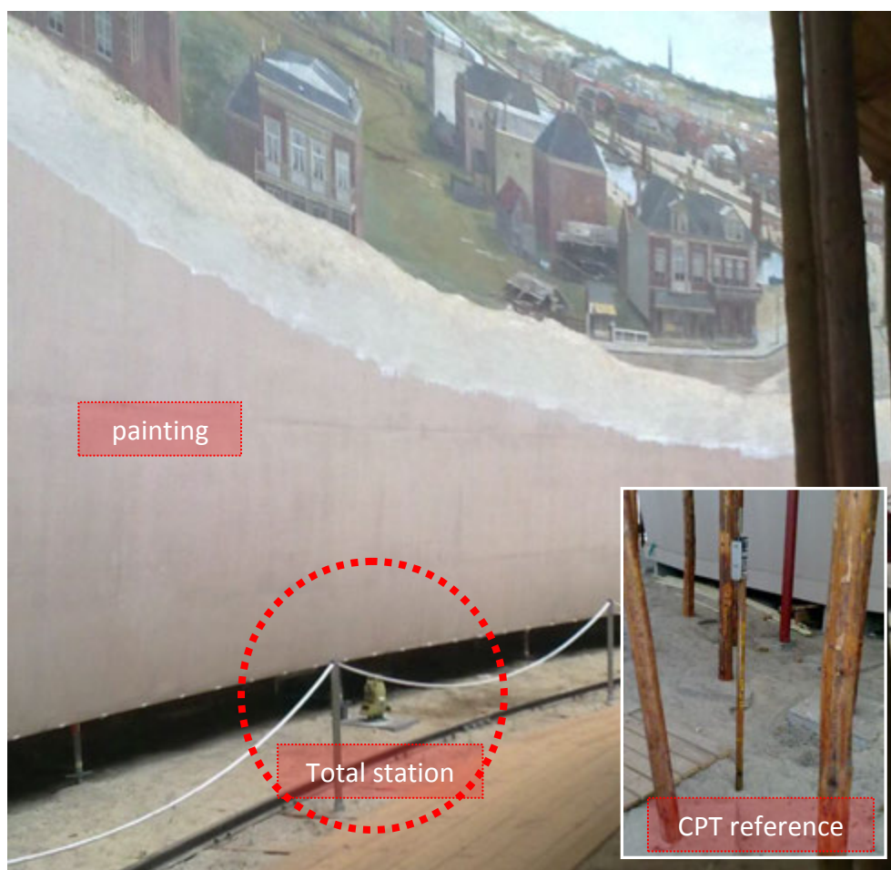
Figure 5b: Total station at foundation level and part of Mesdag's painting ; detail: deep CPT for absolute reference level
