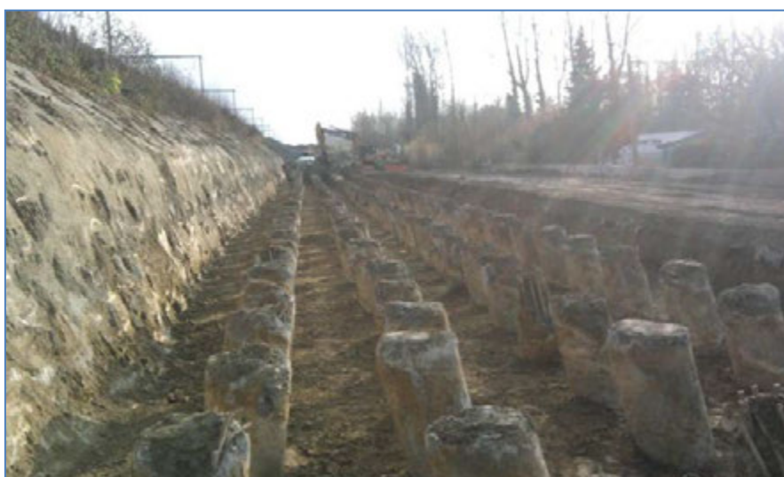
Photo 1: Excavated pile heads and soil nailed wall
