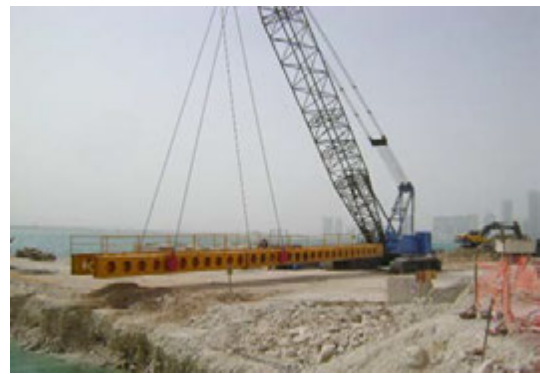
Photo 4: Cantilevered Platform Carried by Crane
