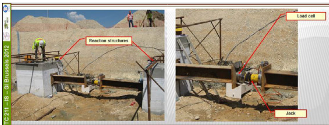
Figure 14: Horizontal full scale load test: reaction structure and load applying system.
