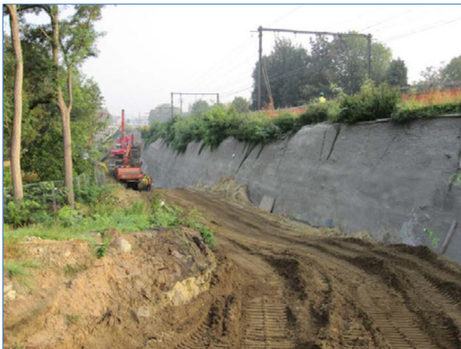
Photo 6: Finished soil nail wall
