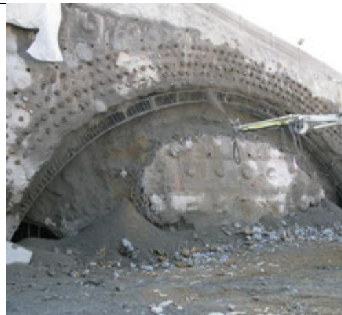
Figure 13: top cavern excavation
