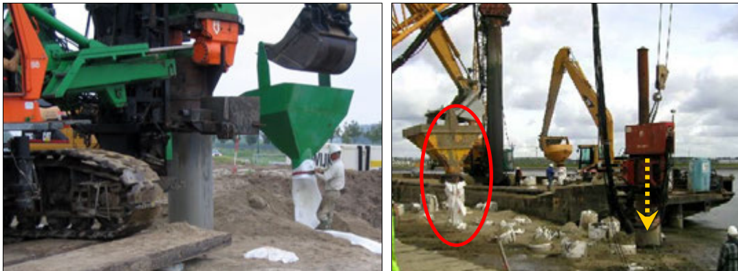
Figure 8: Installation of geotextile encasement (displacement method)
