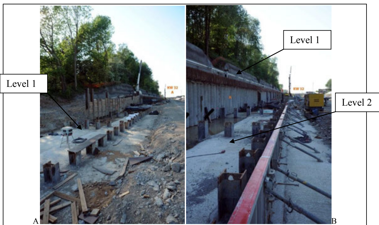
Photo 3: the longitudinal and transversal pile walls put in place
