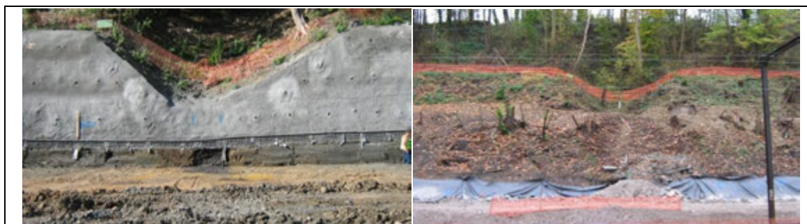
Photo 2: View on the vertical trenches – anno 2009
