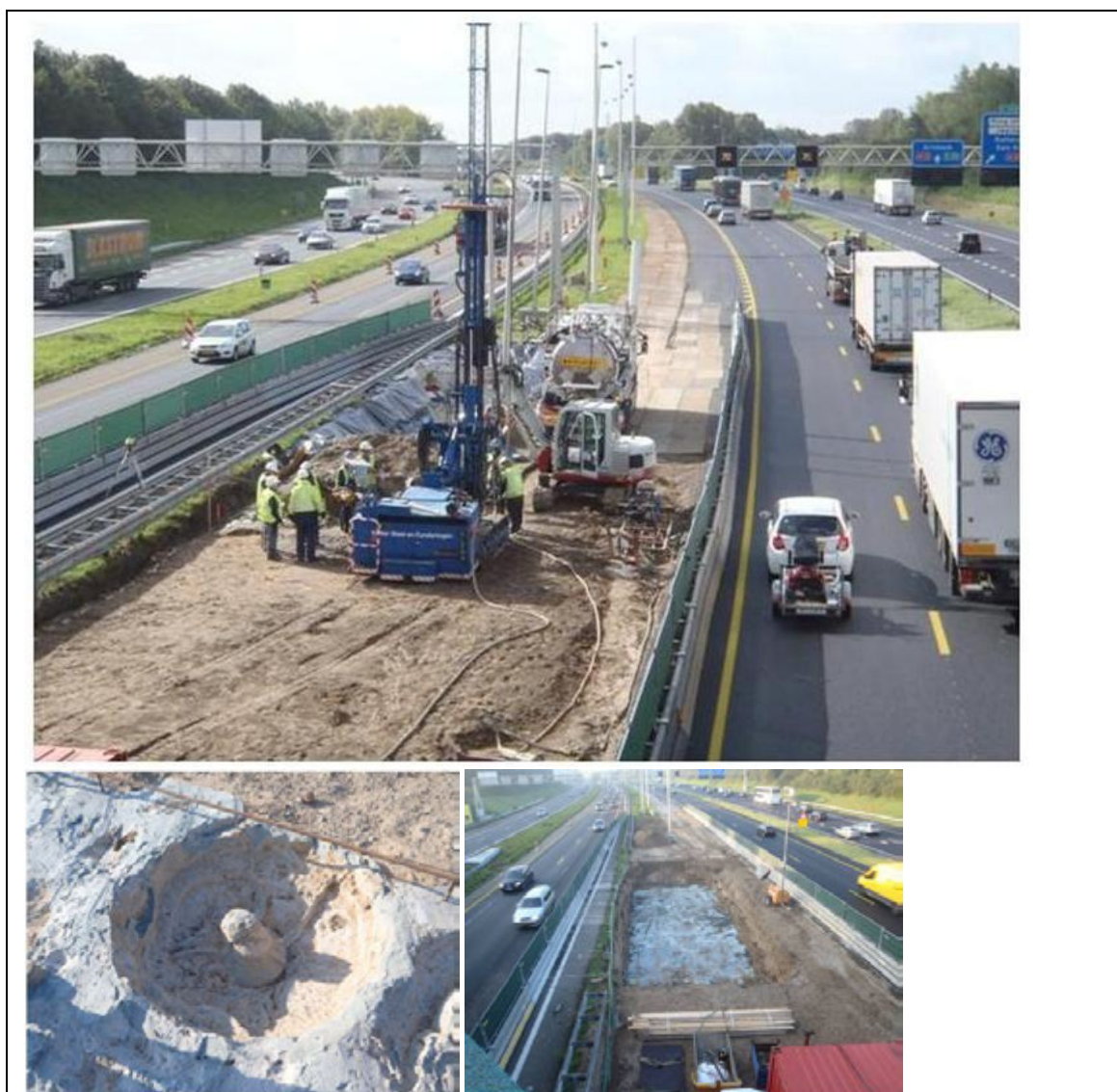
Photo 4: An impression of the execution operations at the centre pillar
