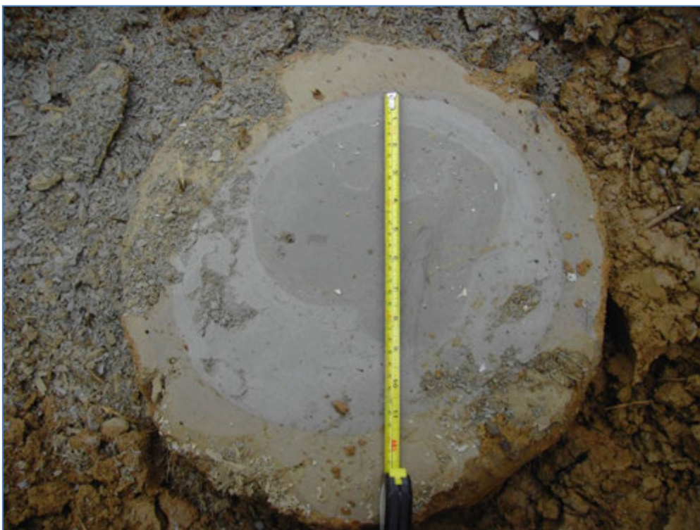
Photo 5: Cross-section of excavated VHP grout nail of 30 cm diam
