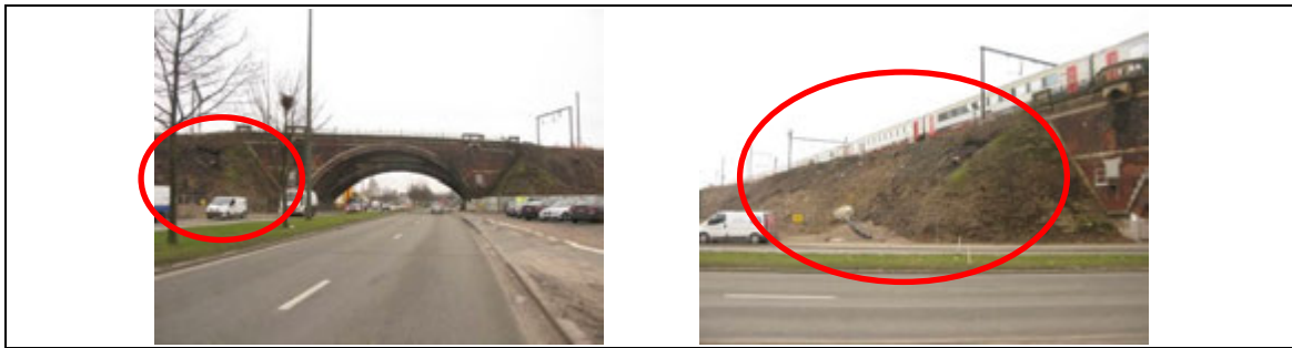
Photo 1: Pictures of the local situation prior to installation
