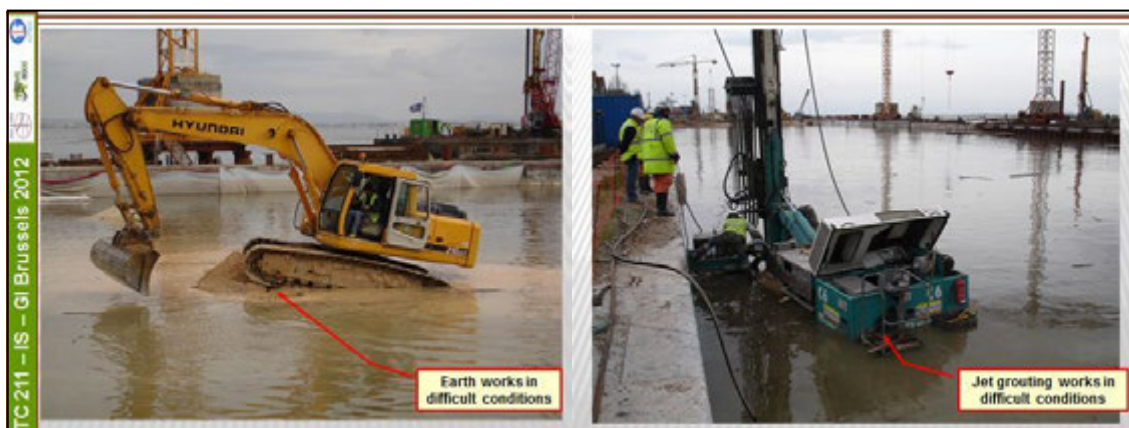
Figure 11: Views of the complex works inside the dockyard.
