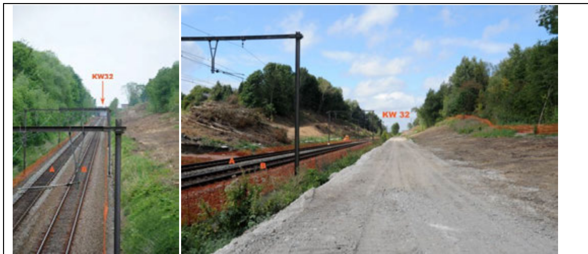
Photo 1: View on the existing situation – anno 2009
