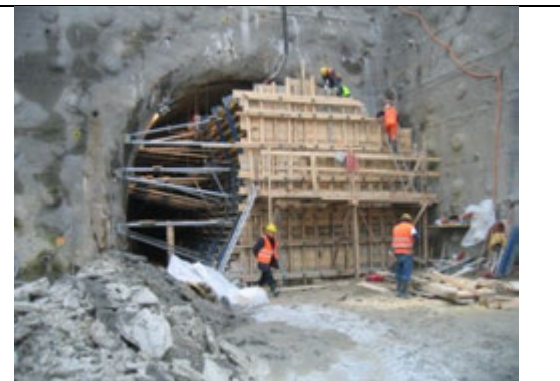
Figure 11: construction of the 48 meters long concrete beams inside the tunnels
