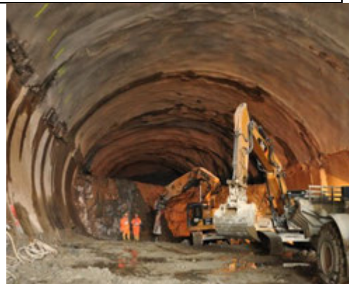
Figure 15: cavern bench excavation
