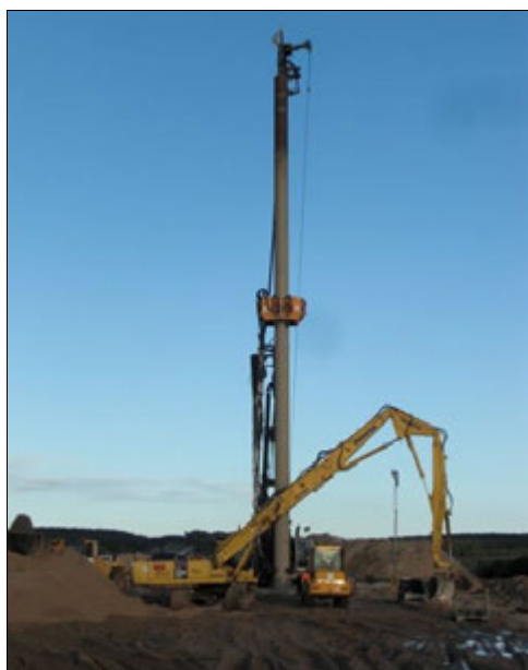
Figure 15: LRB 255 rig with 30 m long displacement pipe on construction site in Poland
