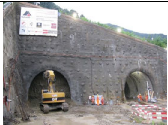
Figure 7: Excavation of the 2 side tunnels
