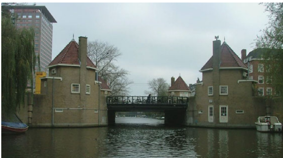
Figure 1: Bridge 404 looking east
