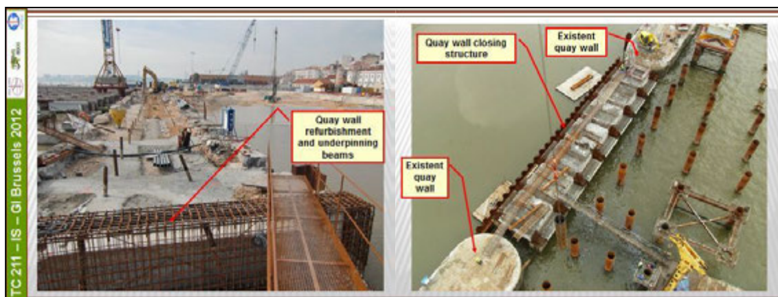
Figure 6: Quay wall underpinning and refurbishment works.
