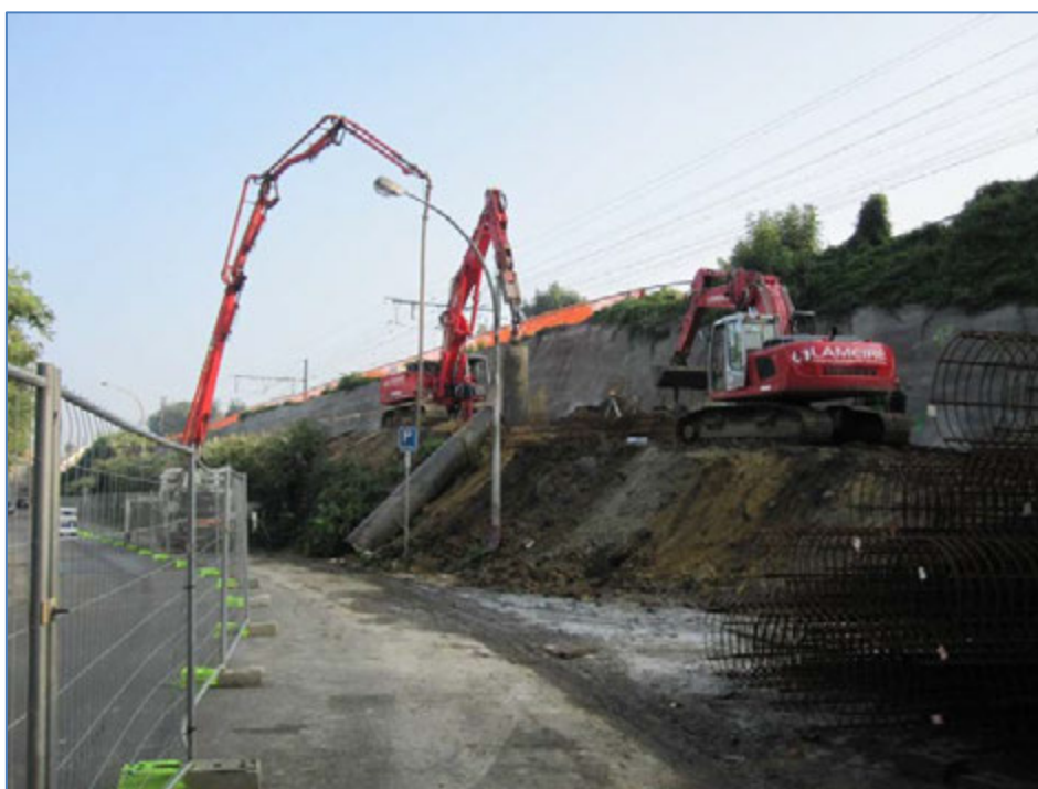
Photo 7: Execution of shaft foundations
