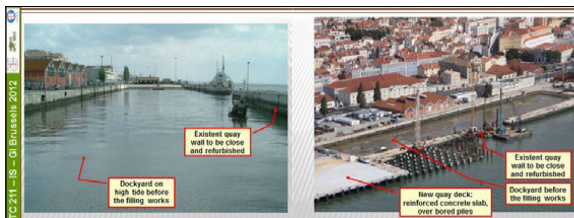
Figure 3: View of the dockyard before the filling works.
