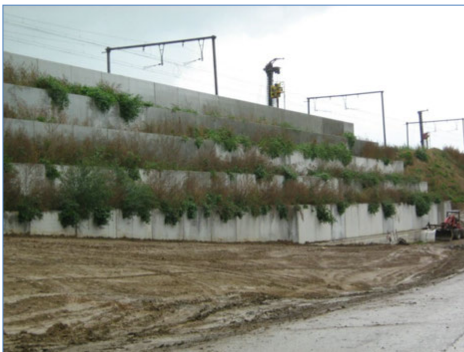
Photo 2: Finished green terrace, with temporary wild vegetation
