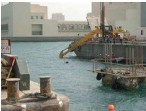
Photo 3: Jet Grouting on Spud-Barge
