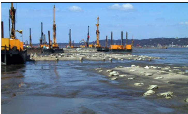
Figure 1: Installation of GEC from pontoons in extremely soft mud
