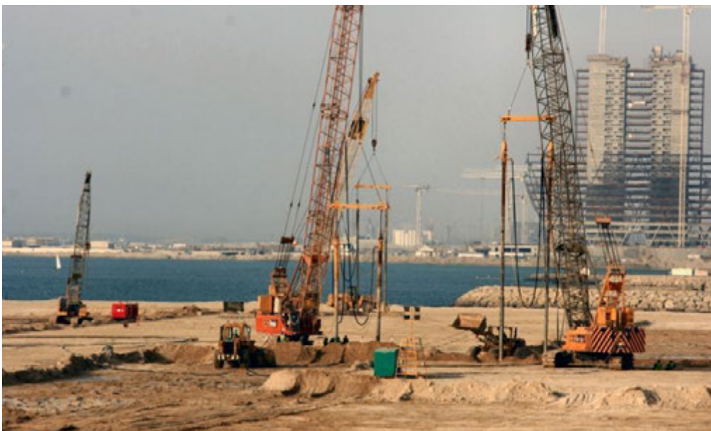
Figure 17 : Vibrocompaction with vibrators in tandem configuration (Keller group).
