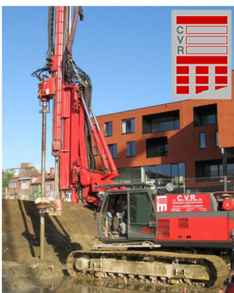
Figure 6: The CVR C-mix® single auger system (available tool diameter for single shaft ranging between 43 and 103 cm), after Denies (2012) , with the courtesy of CVR nv
