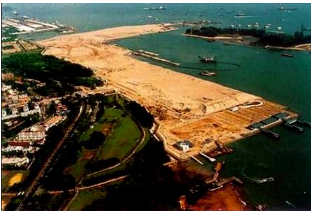
Figure 48: Construction of a new PSA Container Terminal at Pasir Panjang, Singapore
