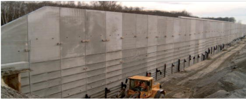
Photo 1: Back view of full height concrete facing with polymer geogrid attachments
