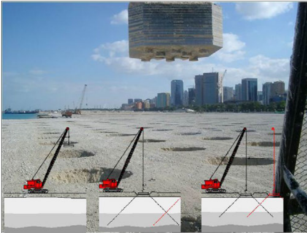
Figure 14: Carrying out of Dynamic Compaction (Menard Group).
