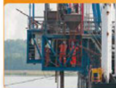
Drilling and blasting
