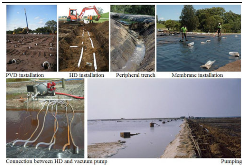
Figure 32: Site preparation for Vacuum consolidation (Courtesy from Austress-Menard)
