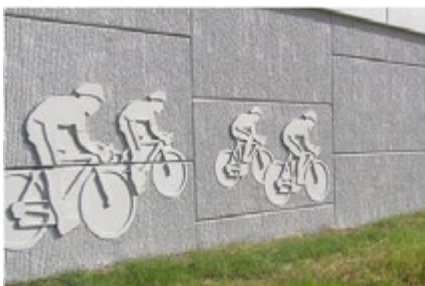
Photo 2: Bicycle artwork on prefabricated concrete facing
