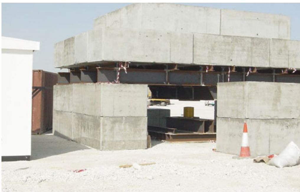
Figure 59: Typical zone load test set-up
