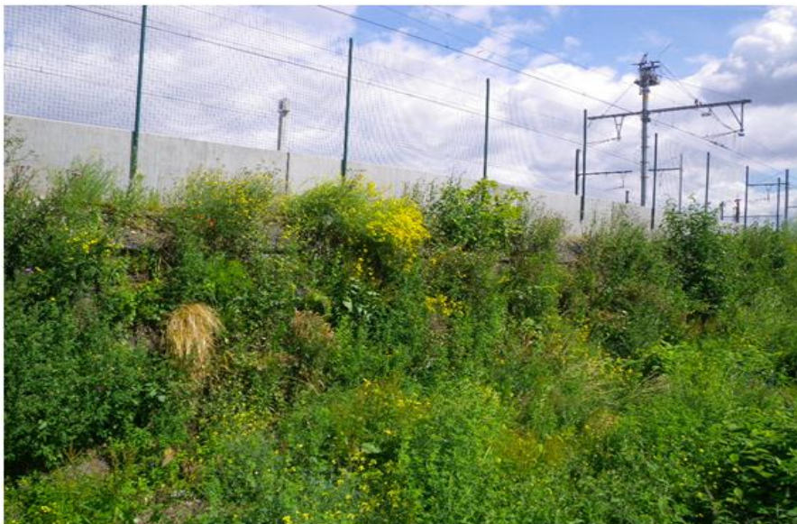
Photo 3: Wrap-around MSE wall with geosynthetic reinforcement
