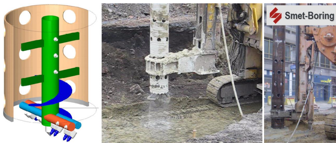
Figure 9: Smet Tubular Soil Mixing TSM system (column diameter of 38 to 73 cm), after Denies (2012) and Topolnicki (2012) with the courtesy of Smet-Boring nv
