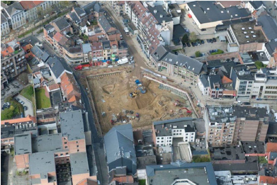
Figure 46: Excavation in the downtown of Aalst (Belgium), after Leemans (2012)
