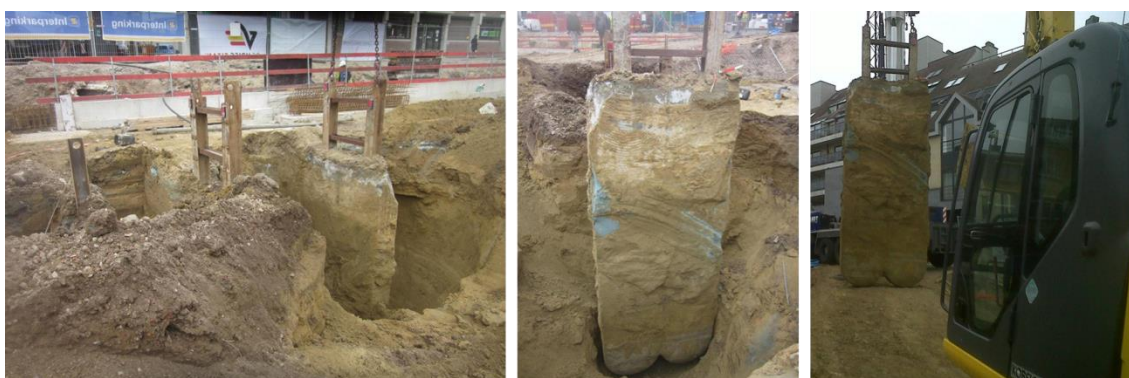
Figure 50: Excavated extra CSM panels for mechanical characterization, after Leemans (2012)
