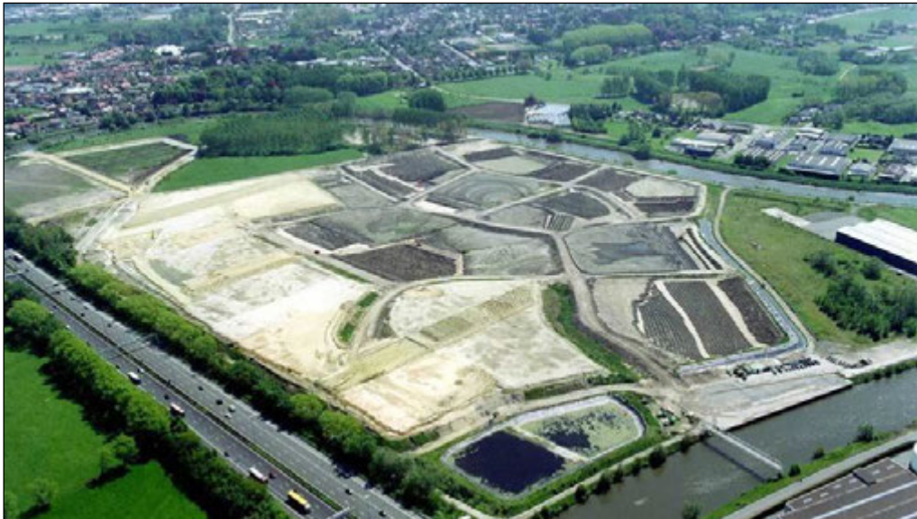
Figure 52: Lagooning at FASIVER site, Zwijnaarde, Belgium
