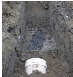
Foundation segments to support sewage pipes
