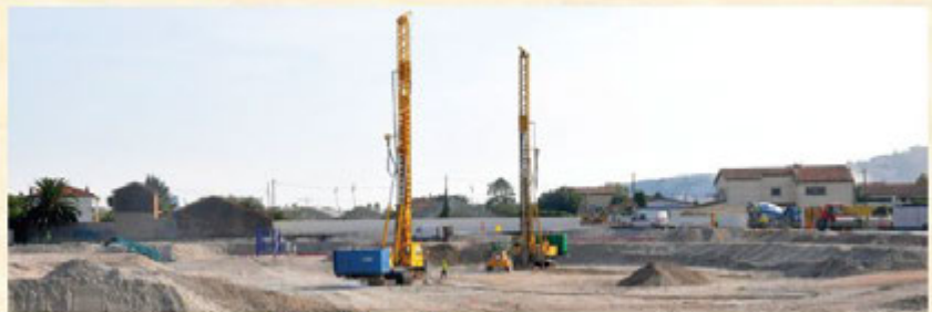
Ecostadium de Nice (vibrocompactage)
