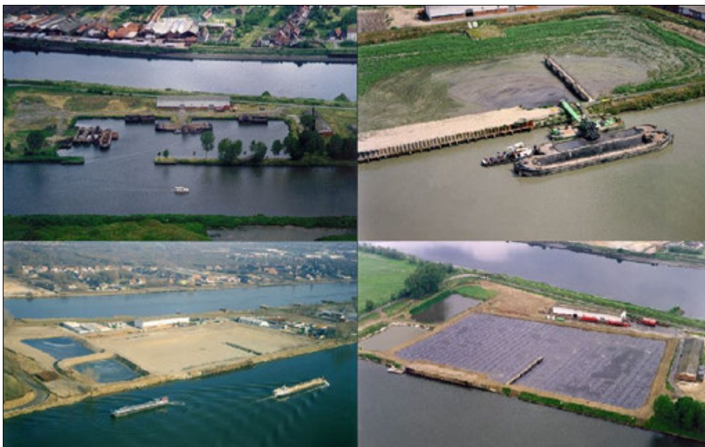
Figure 34: Project at Ruisbroek; successful application of vacuum consolidation technique
