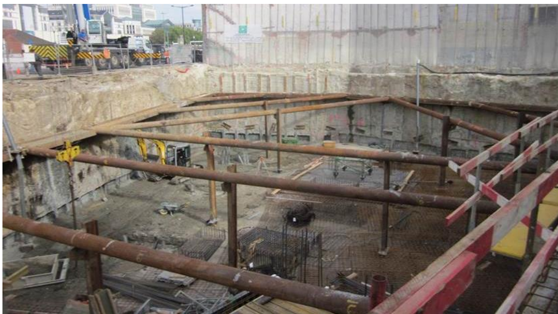
Figure 45: Shored CSM walls in Belgium, after Leemans (2012)
