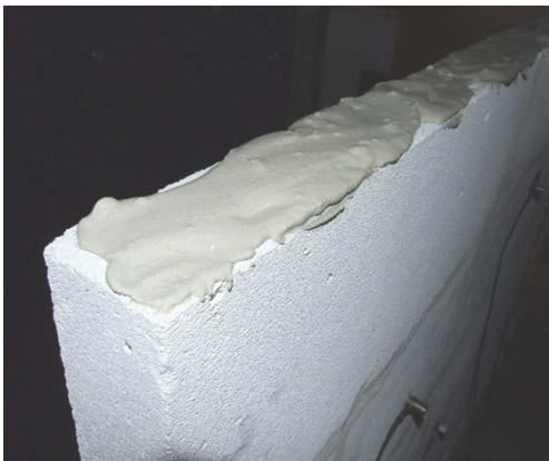
Figure 7: Application of a mortar joint
