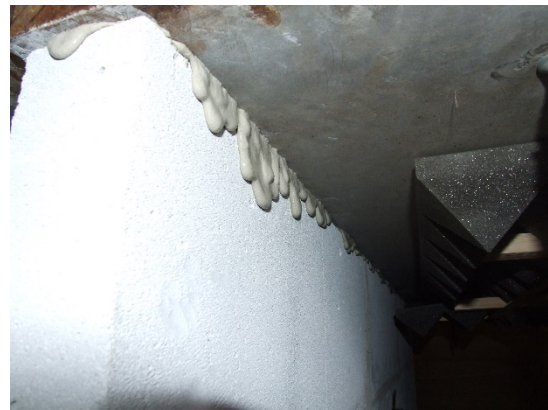
Figure 8: A perfect connection on the whole surface
