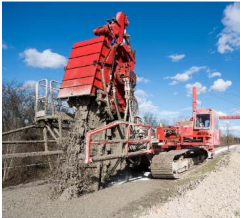
Fig. 17. Trenchmix system of Soletanche-Bachy/Mastenbroek used for the realization of soil mix wall in one single continuous pass (with the courtesy of Soletanche-Bachy)
