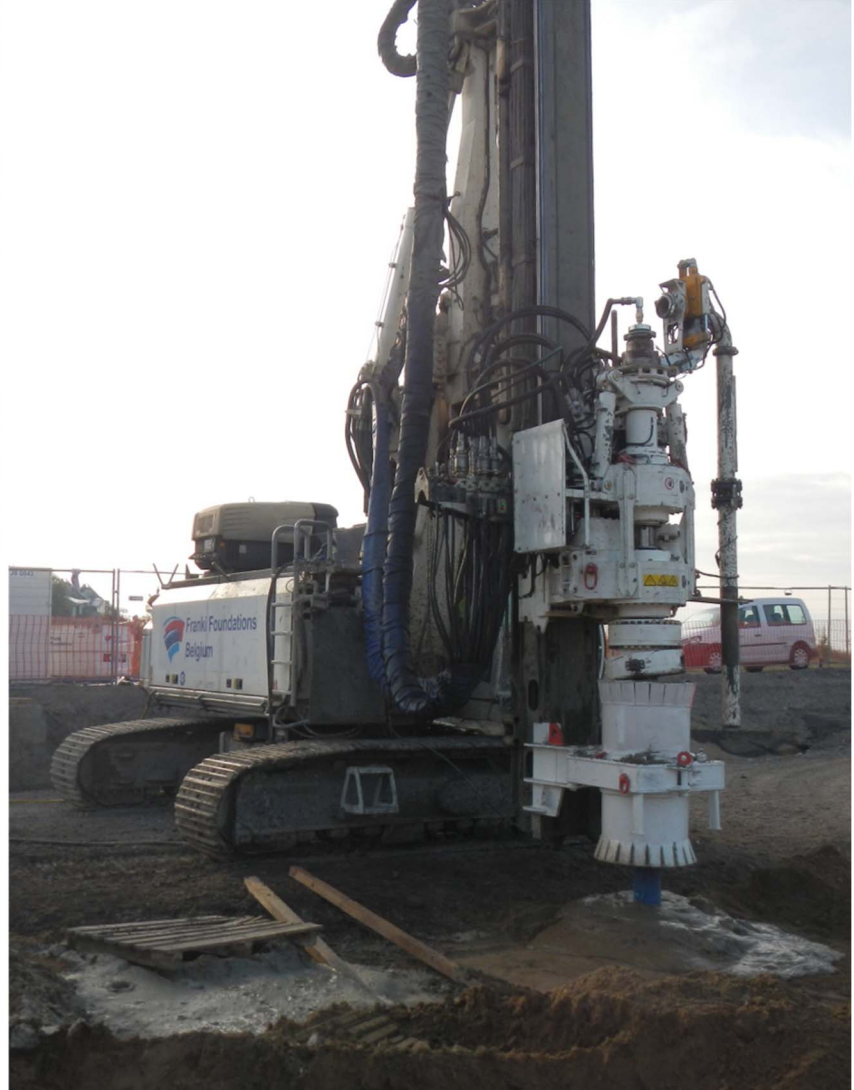
Fig. 9. Execution of secant soil-cement columns with an ABI drilling/mixing head – execution in single shaft configuration (with the courtesy of Franki Foundations – group Besix)
