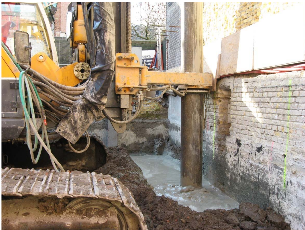
Fig. 24. Execution of a soil mix wall (CSM technique) along existing foundations
