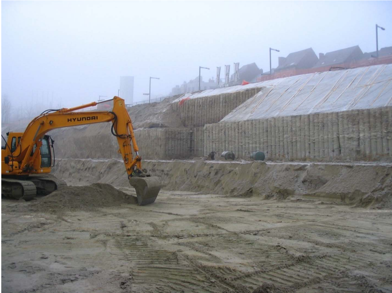
Fig. 25. Execution of a soil mix wall along an existing slope
