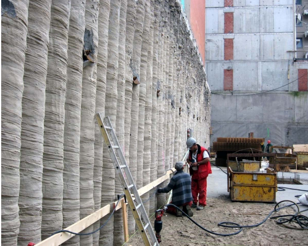
Fig. 3. Enlarged view of an anchored soil mix wall (made with the CVR C-mix® technique) used as retaining structure for the realization of an excavation (with the courtesy of CVR nv)
