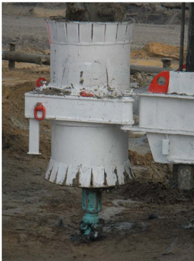
Fig. 9. Execution of secant soil-cement columns with an ABI drilling/mixing head – execution in single shaft configuration (with the courtesy of Franki Foundations – group Besix)
