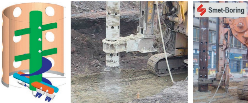
Figure 11.5 Smet Tubular Soil Mixing TSM system (column diameter of 38–73 cm). (Source: After Denies et al. (2012a) and Topolnicki (2012) , with courtesy of Smet-Boring nv).
