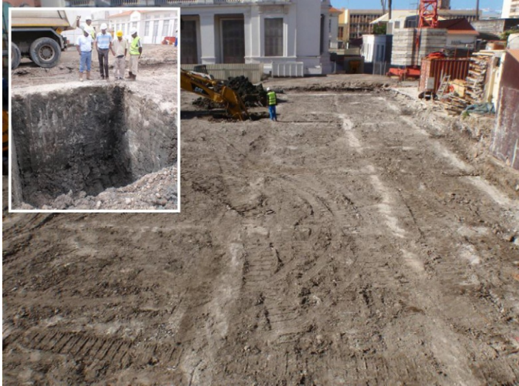
Figure 11.16 Arrangement of the Geomix caissons made of CSM panels. (Source: After Benhamou and Mathieu (2012) , with courtesy of Soletanche Bachy ).
