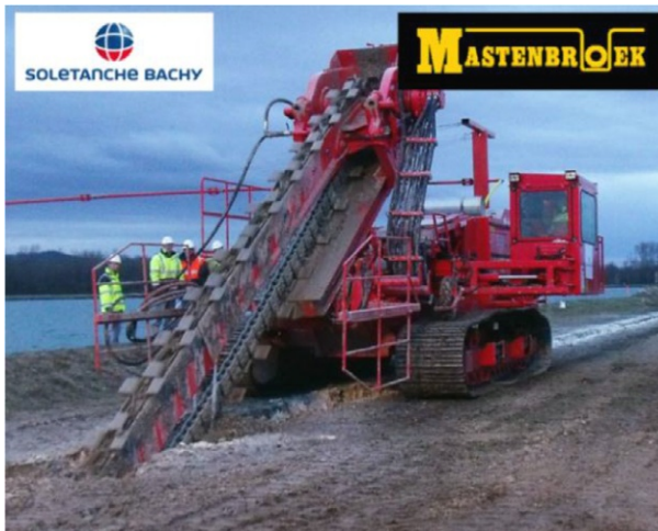
Figure 11.8 Trenchmix tool. (Source: Courtesy of Soletanche-Bachy/Mastenbroek).
