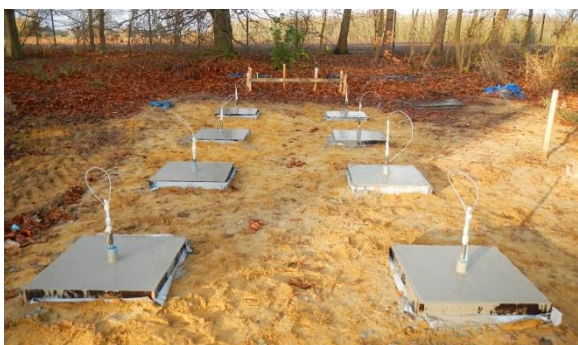
Figure 6. Test location after concreting the eight slabs
