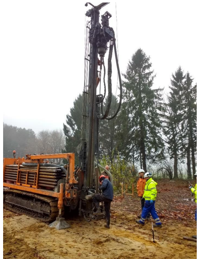
Figure 3. Dry drilling of the steel bars into the ground
