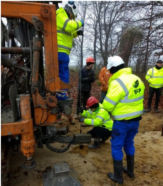
Figure 4. Installation of the injection tube inside the hollow steel bar
