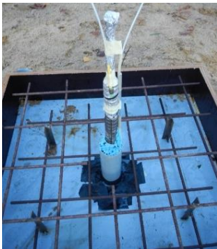
Figure 5. Isolation of the steel bar with the PU foam
